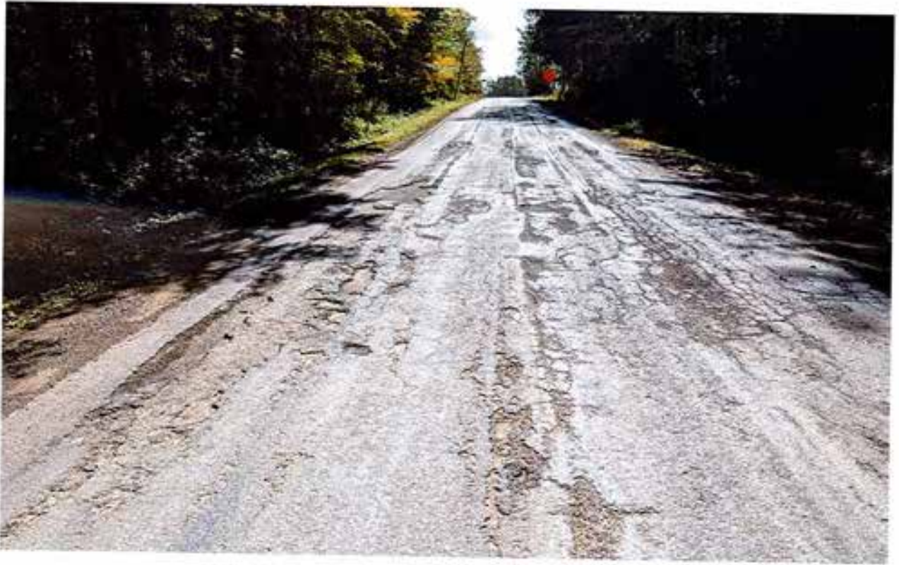
Galen Hill Road lane from Phillippi Rd to 10553
