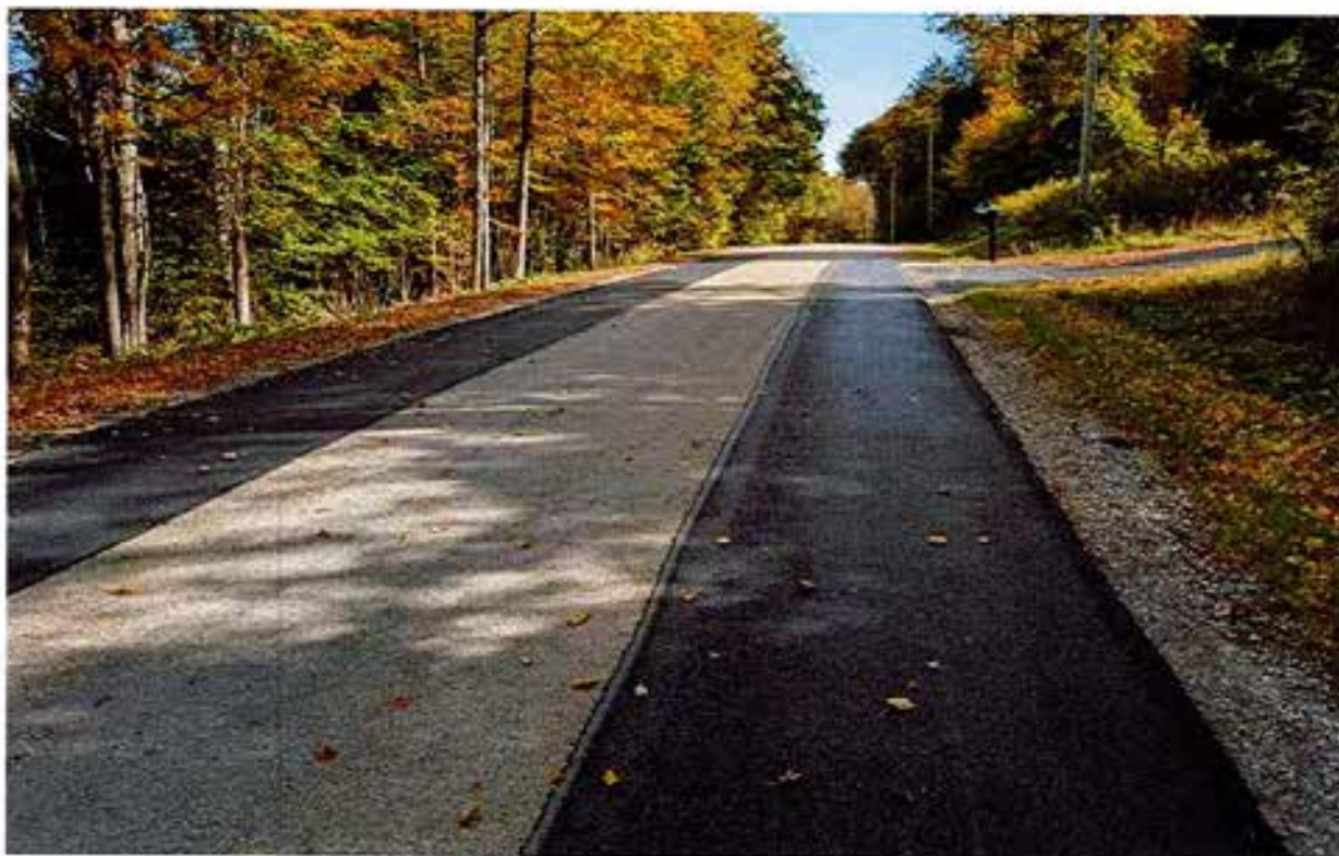
Eagle Street lane and edge near 931 (REPAIRED)
