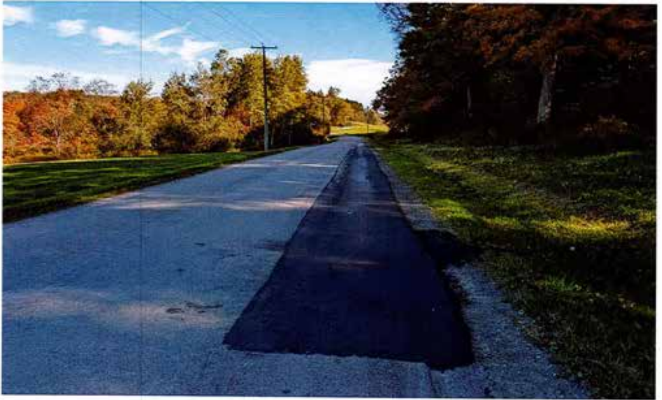
East edge of North Road (REPAIRED)
