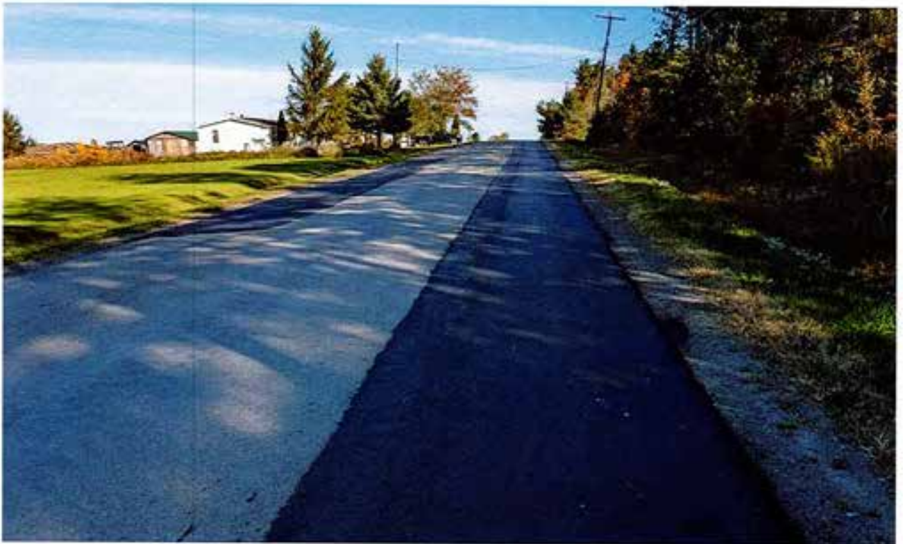
North Road lane and edge South of 11875 (REPAIRED)
