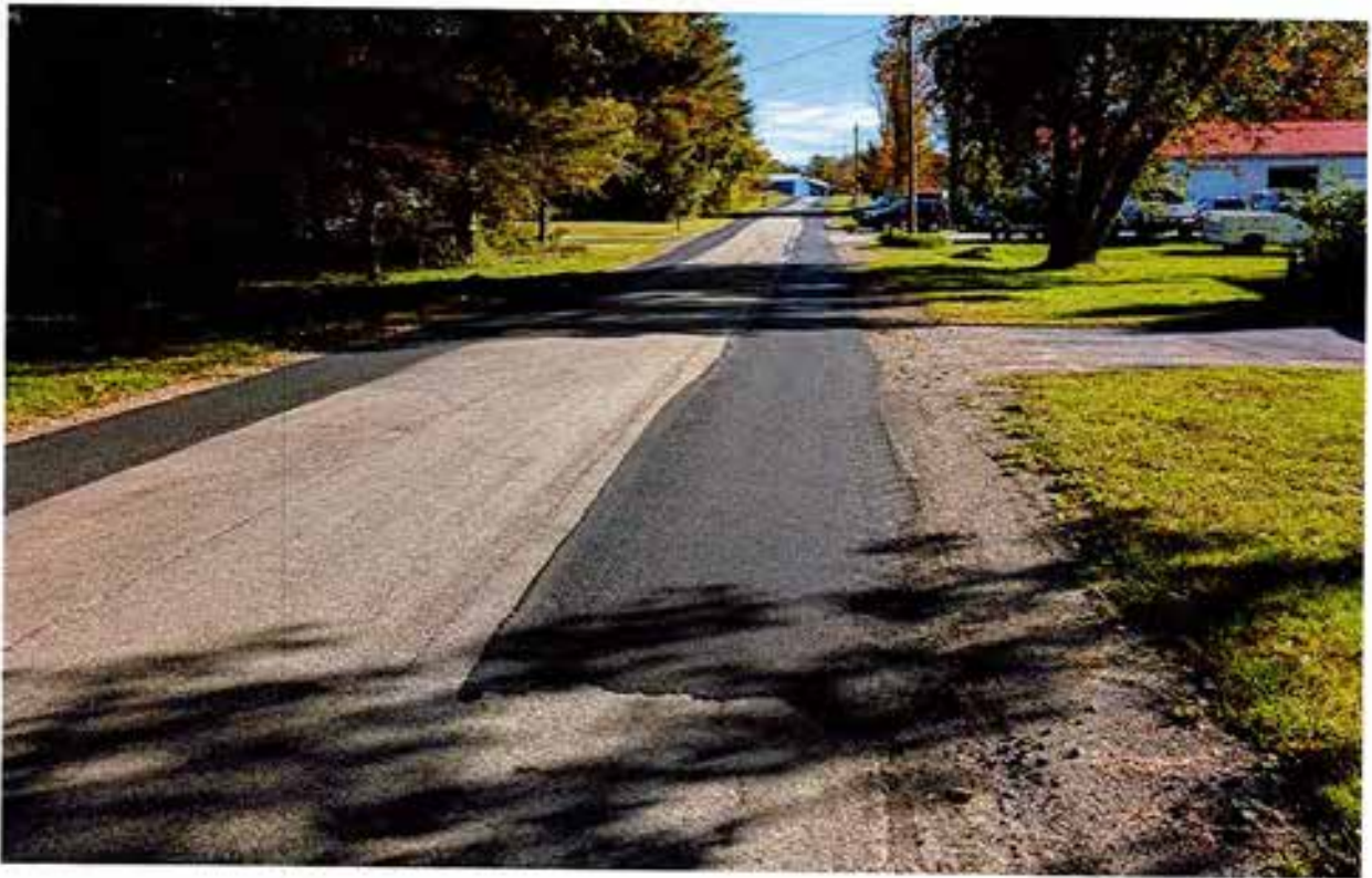
Eagle Street lane and edge near 1253 (REPAIRED)
