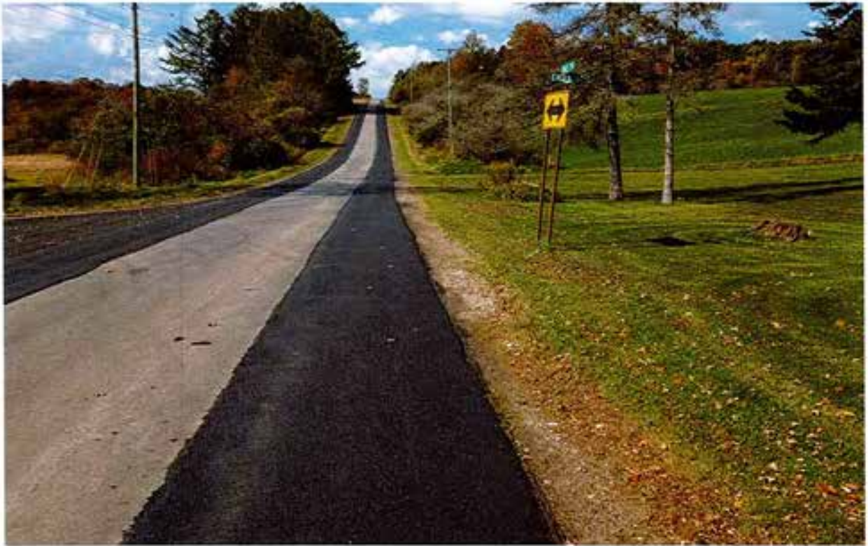
Bray Road Edge at Eagle Street Intersection (REPAIRED)
