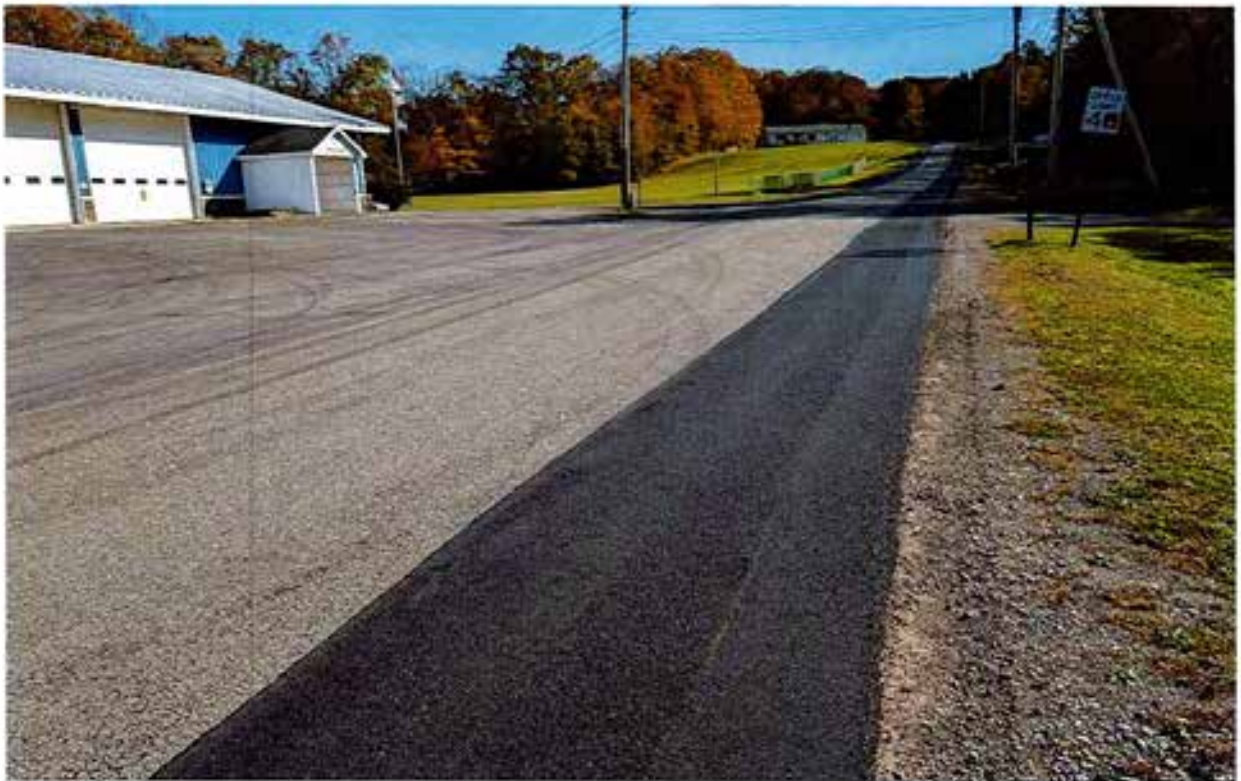
Eagle Street South side lane and edge near 11405 (REPAIRED)
