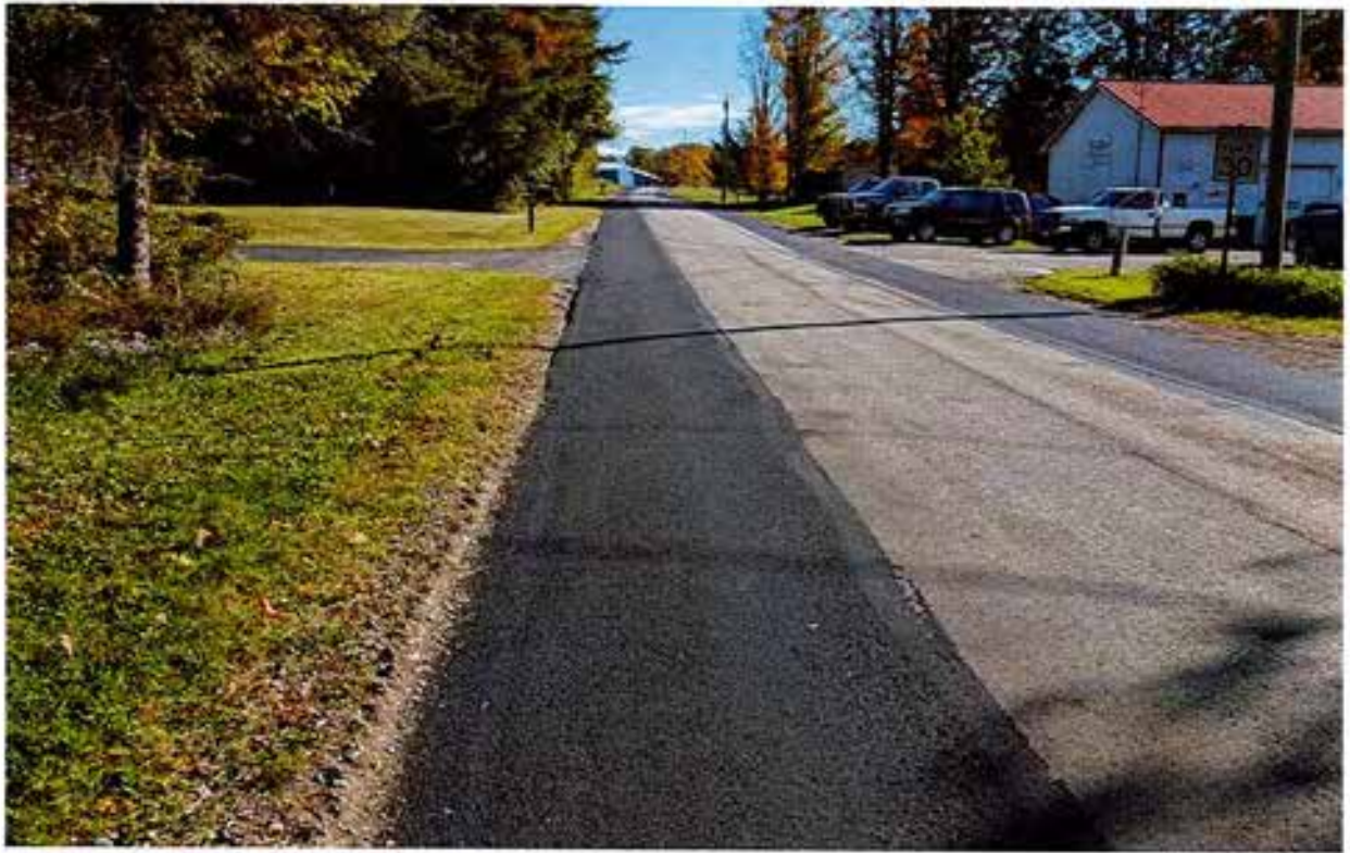
Eagle Street East and West side lane and edge near 1244 (REPAIRED)
