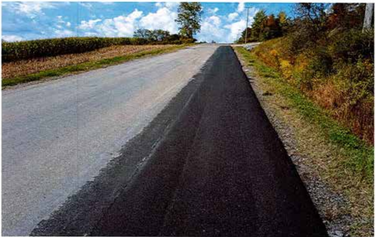
Bray Road lane near 2801 (#2) (REPAIRED)
