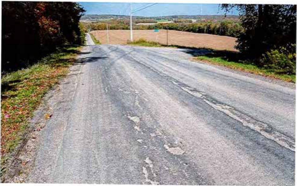
Galen Hill Road intersection with Phillippi Rd lane
