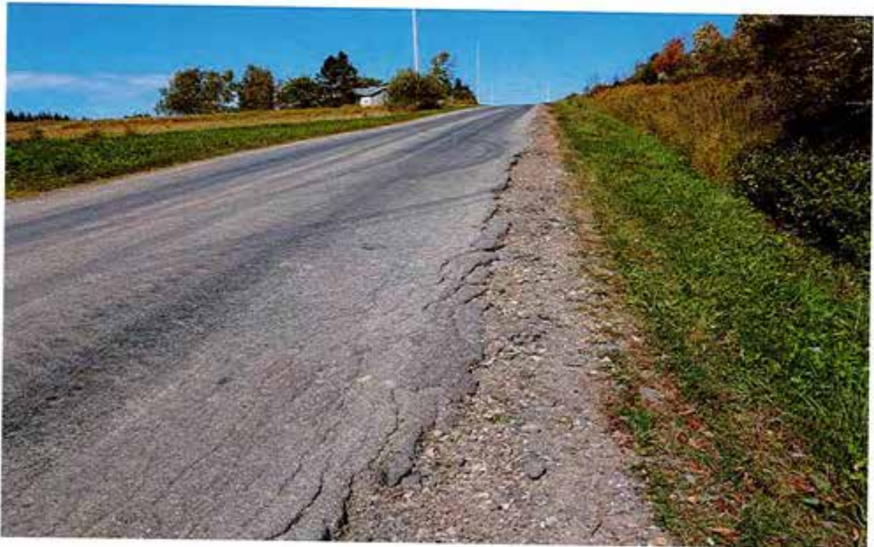
Sandbank Road East edge and shoulder near 9999
