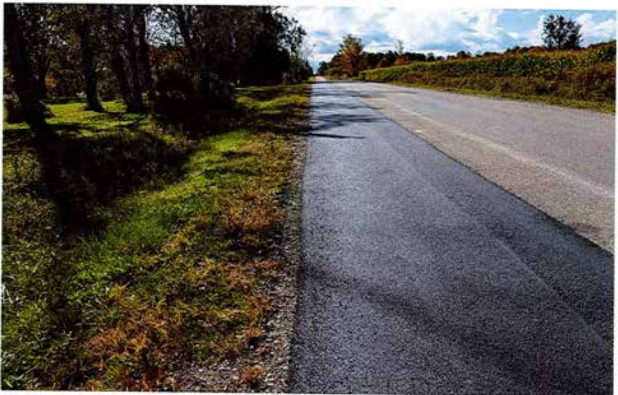
Brown Schoolhouse Road East shoulder South of 11748 (REPAIRED)
