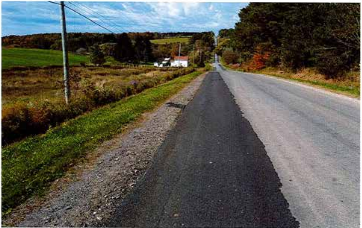
Bray Road South edge and shoulder from 475 to Eagle Street (REPAIRED)
