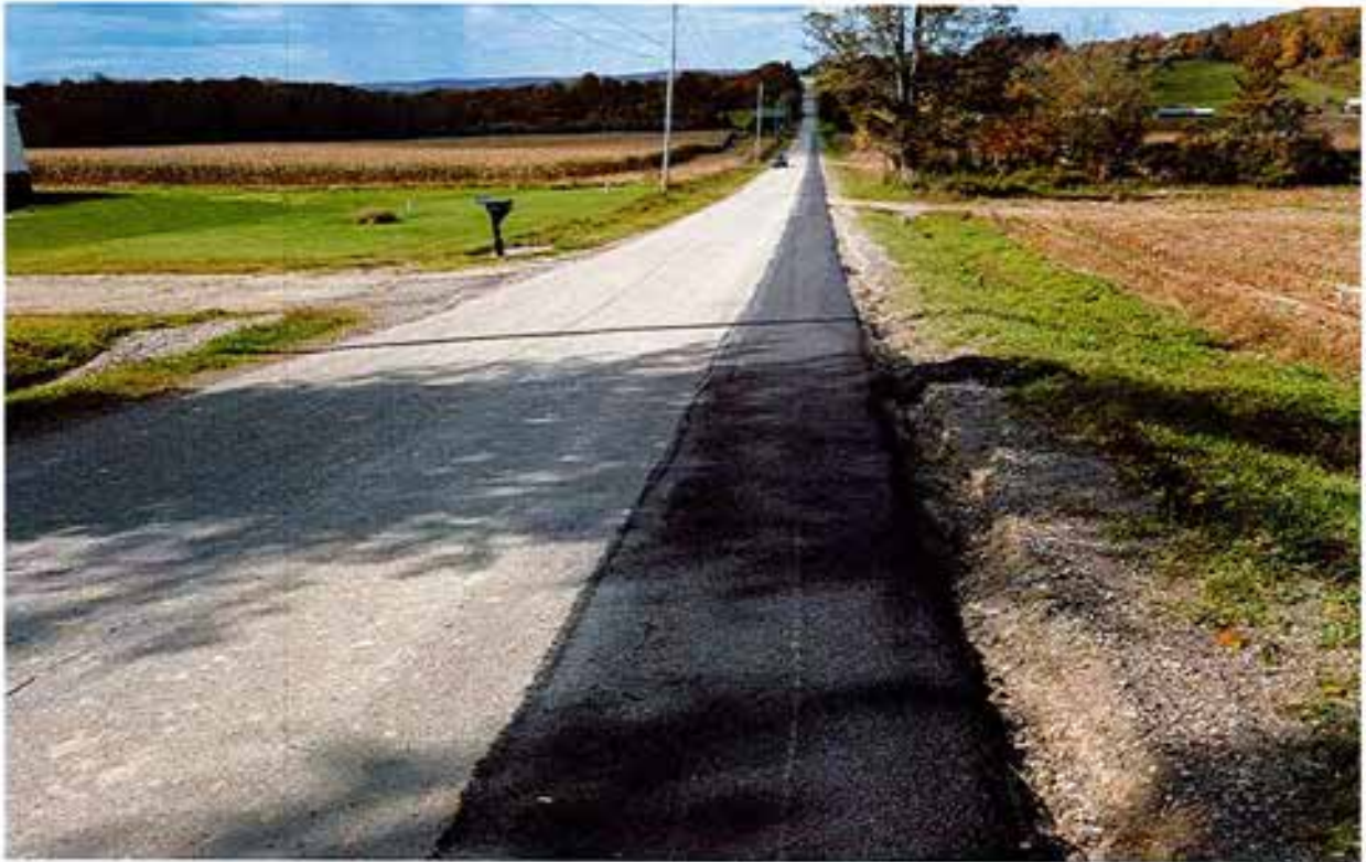
Fisher Blake Road North edge and shoulder near 2195 (REPAIRED)
