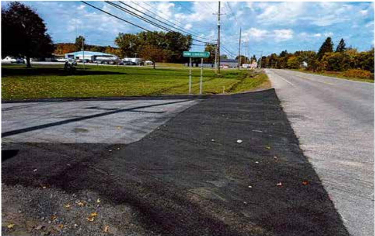
Brown Schoolhouse Road lane near intersection with Route 98 (REPAIRED)
