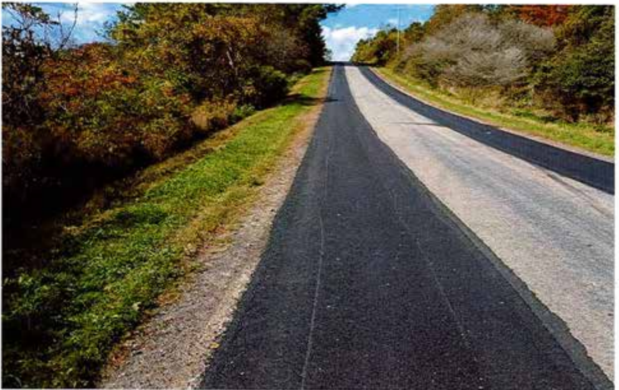
Bray Road South edge and shoulder from Eagle Street to +/- 2801 (REPAIRED)
