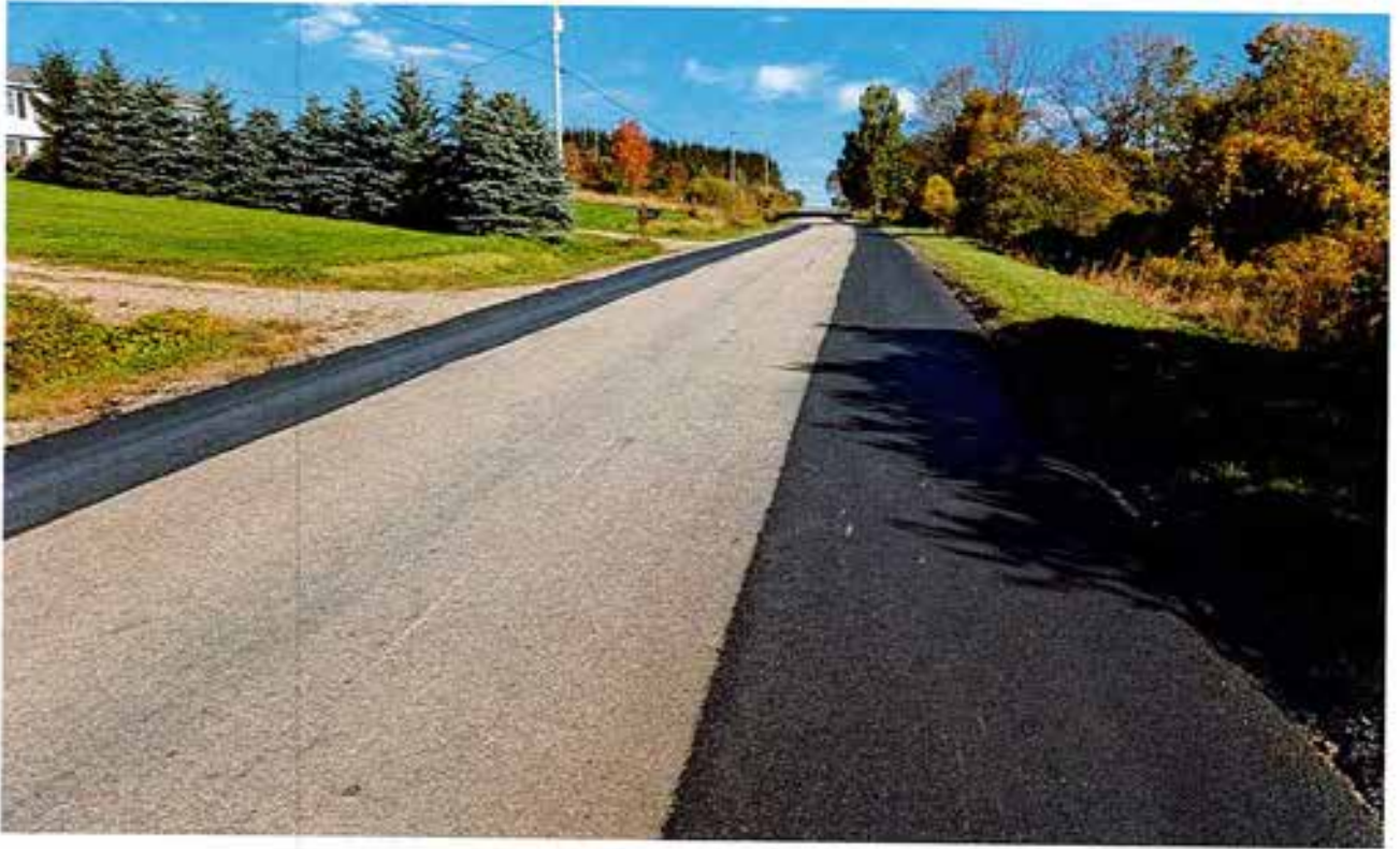
North Road East edge and shoulder near 11509 (REPAIRED)
