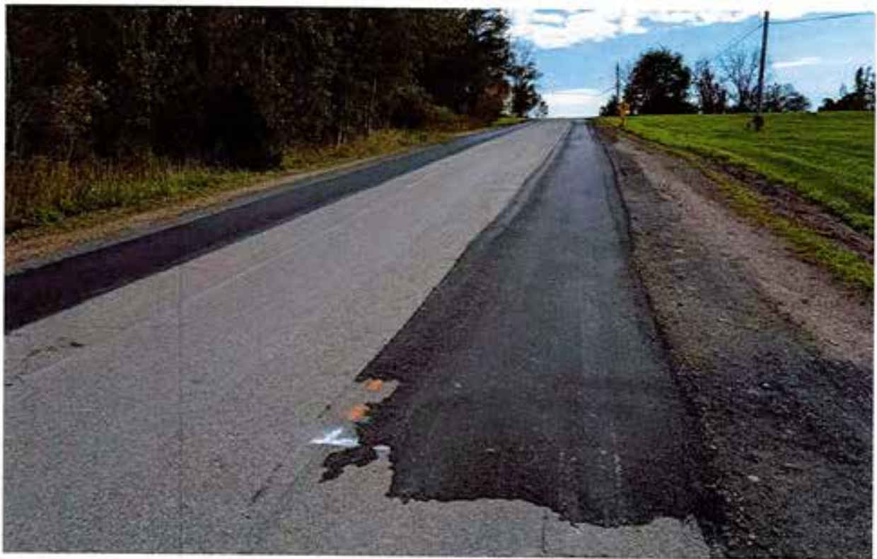
Hughes Road edge and shoulder on North and South sides East of 951 (REPAIRED)
