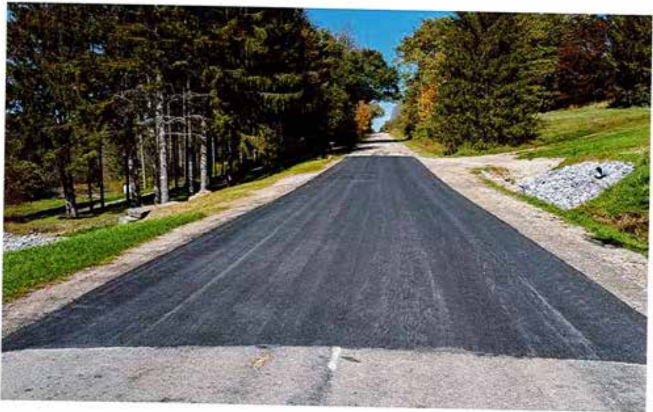
Osmun Rd: Road over Culvert near 10379 facing North (REPAIRED)
