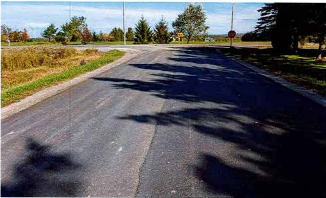
North Rd near intersection with Bray Rd (REPAIRED)
