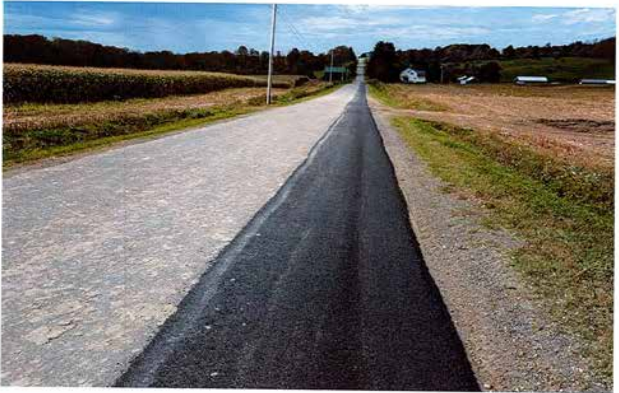
Fisher Blake Road North edge and shoulder from 2195 to +/- 2272 (REPAIRED)
