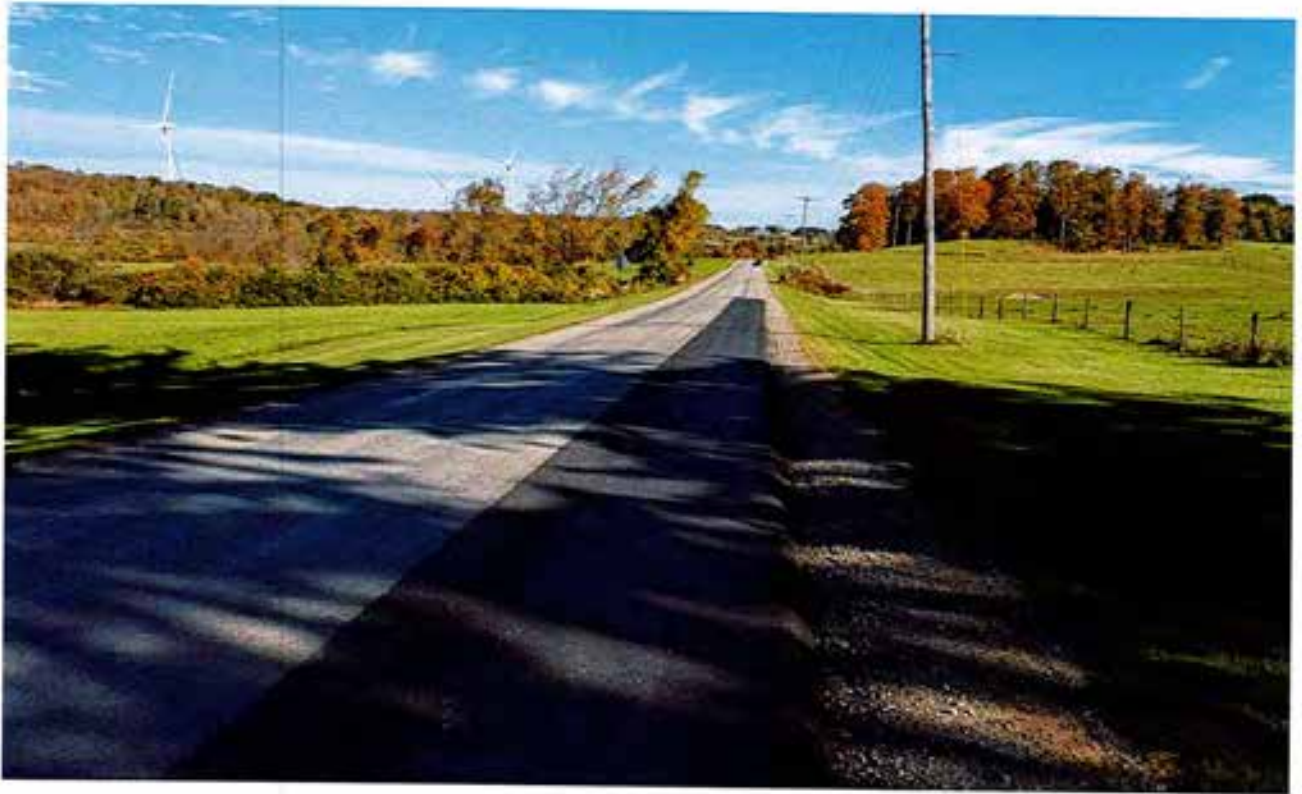
East edge of North Road (REPAIRED)
