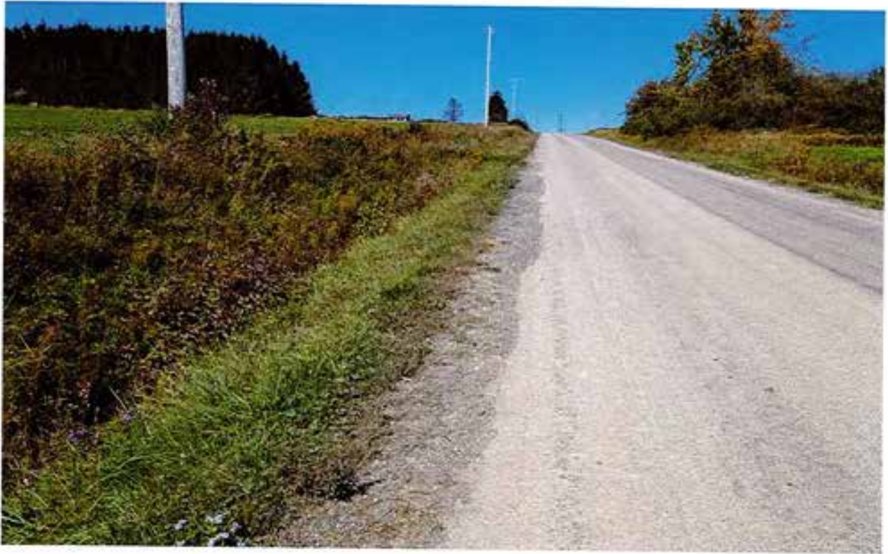
Galen Hill West edge and shoulder North of 10075
