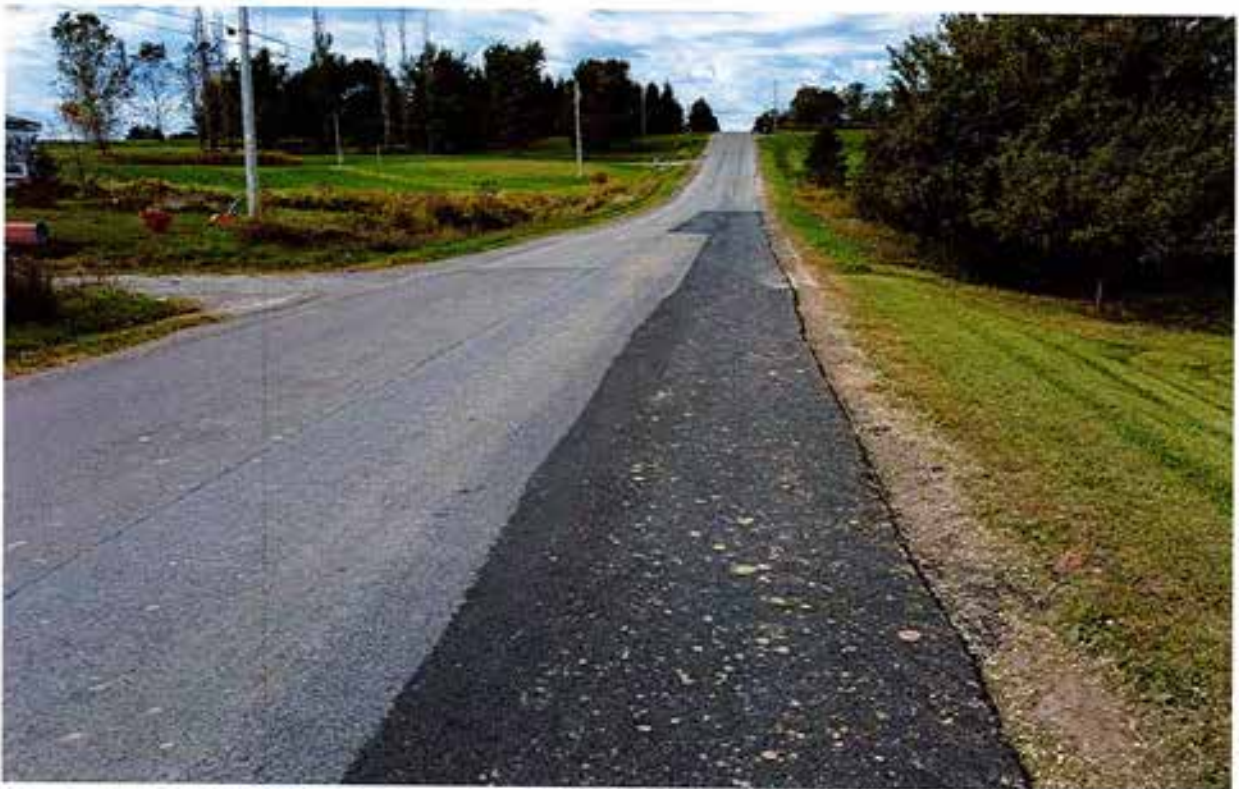
Bray Road North edge and shoulder near 245 (REPAIRED)
