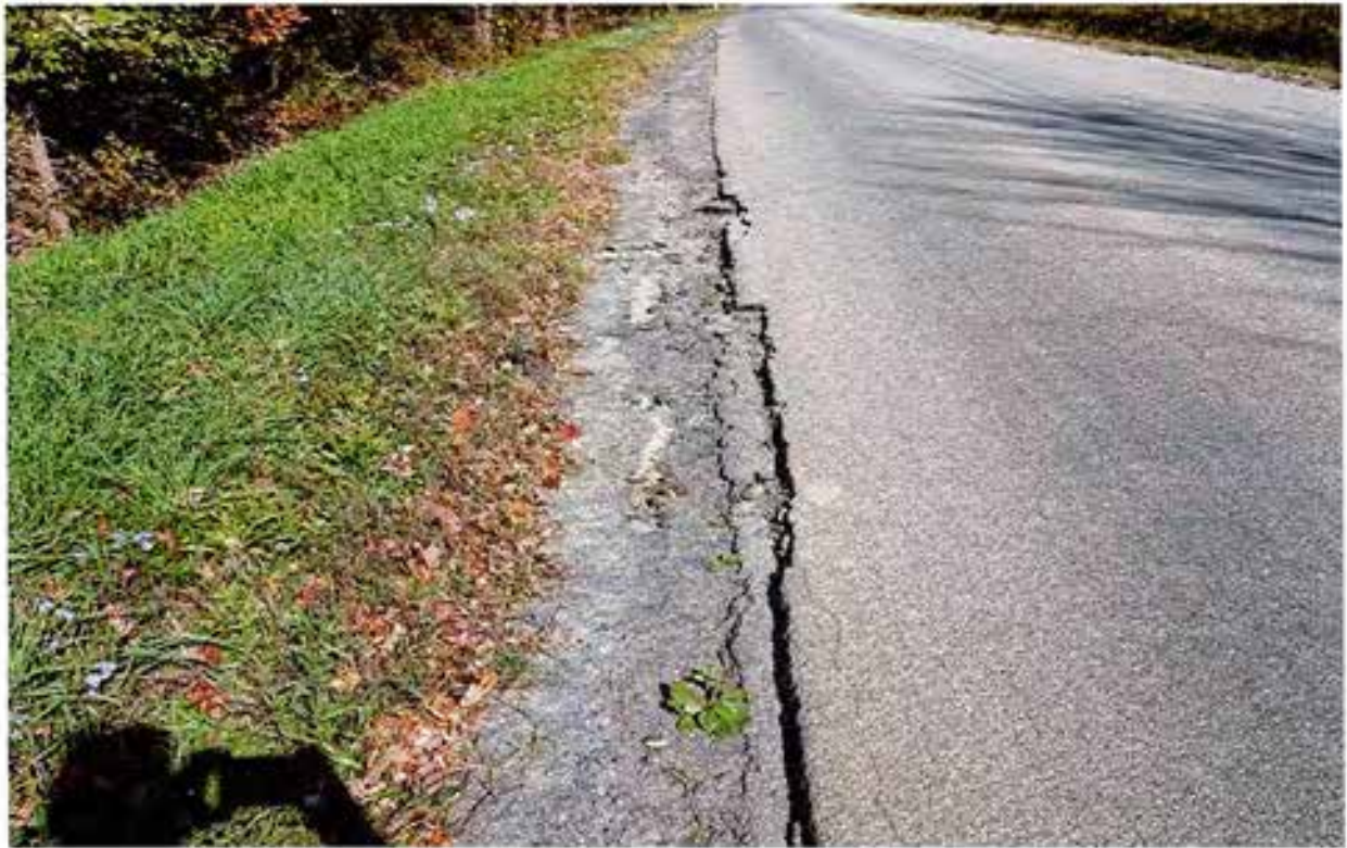
Brown Schoolhouse Road West shoulder North of 11448
