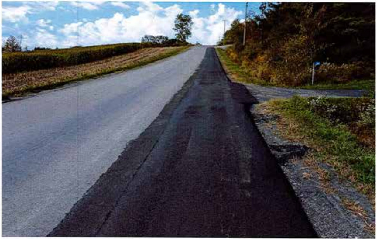
Bray Road North edge and lane near 2801 (#1) (REPAIRED)
