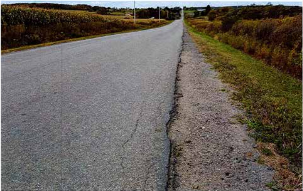
Bray Road North edge and shoulder from gas pipeline #57 to +/- House 113
