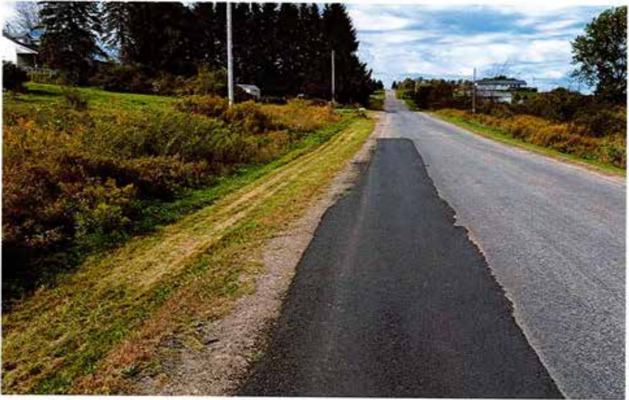
Bray Road South edge and shoulder near 223 (REPAIRED)
