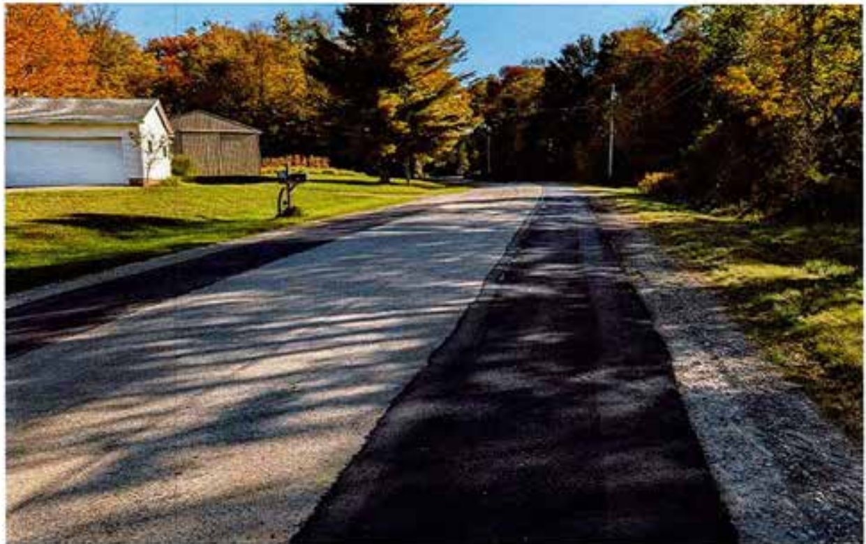
Eagle Street lane and edge near 1152 (REPAIRED)
