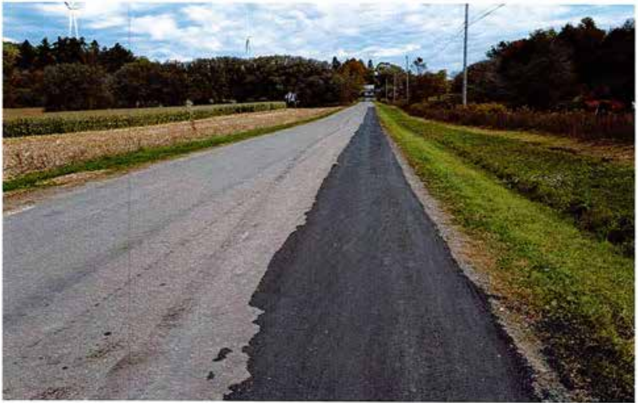
Eagle Street lane and edge North of 757 (REPAIRED)
