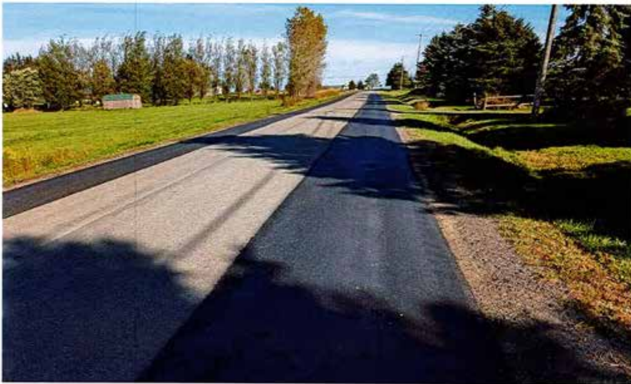
North Road lane, edge, and shoulder near 11980 (REPAIRED)
