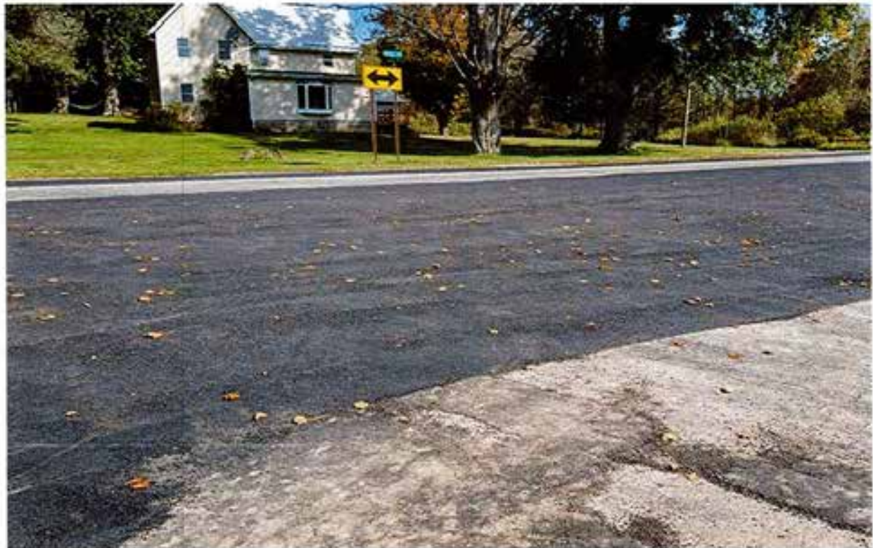
Bray Road lane near intersection with Eagle St (REPAIRED)
