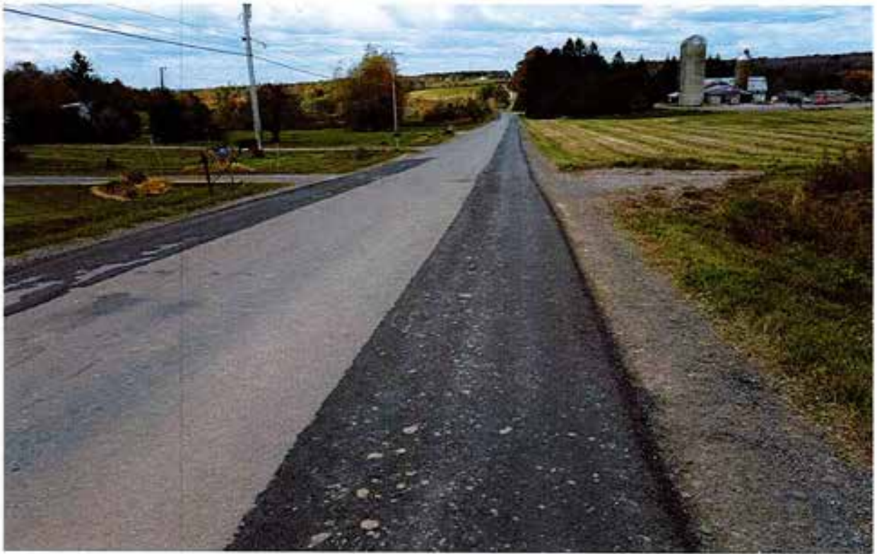
Bray Road North edge and shoulder from 409 to 475 (REPAIRED)
