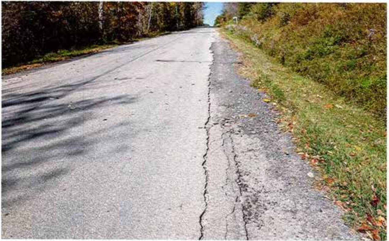
Osmun Rd East side lane, edge, and shoulder North and South of 10410
