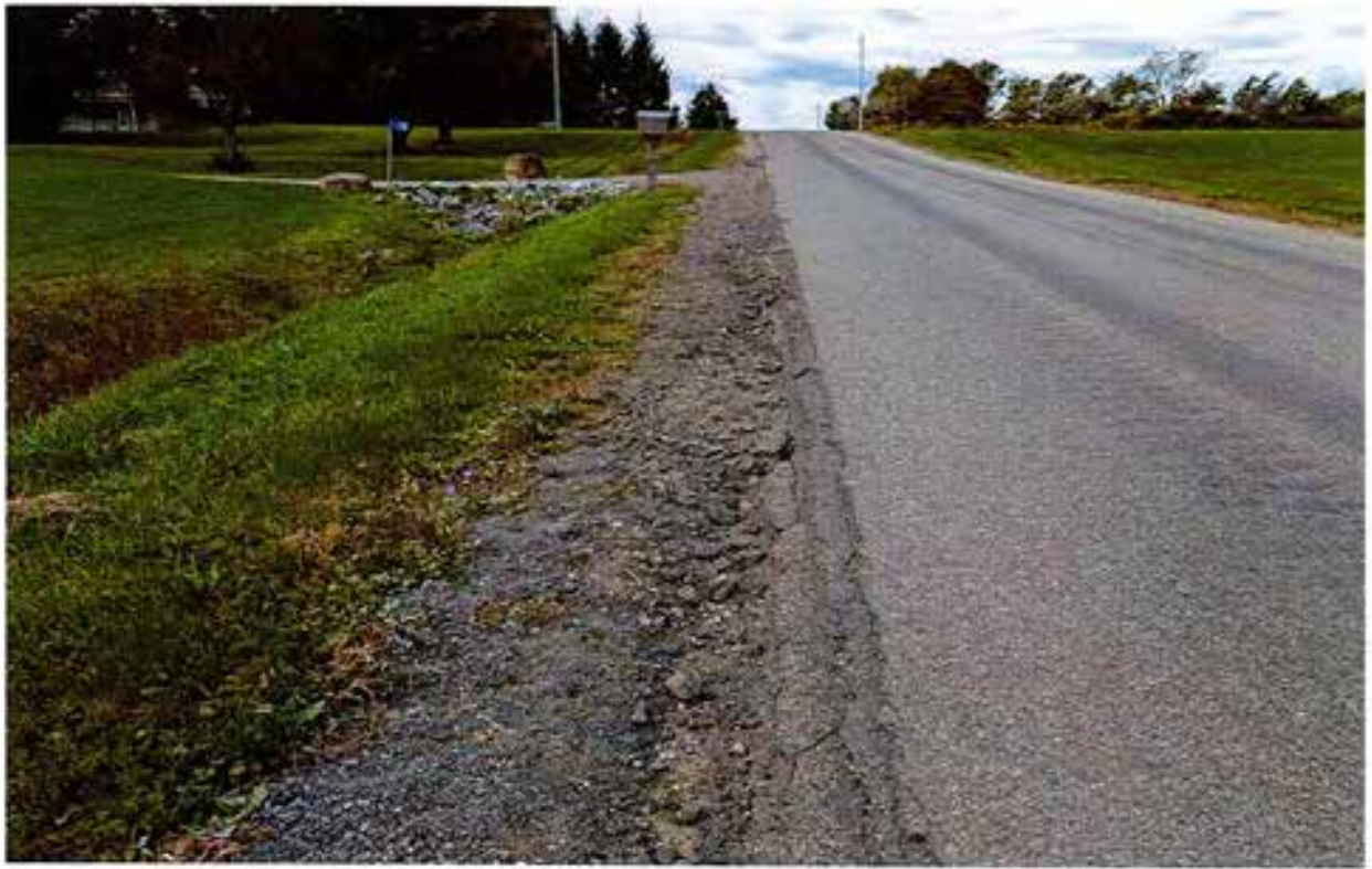
Bray Road South edge and shoulder near 259
