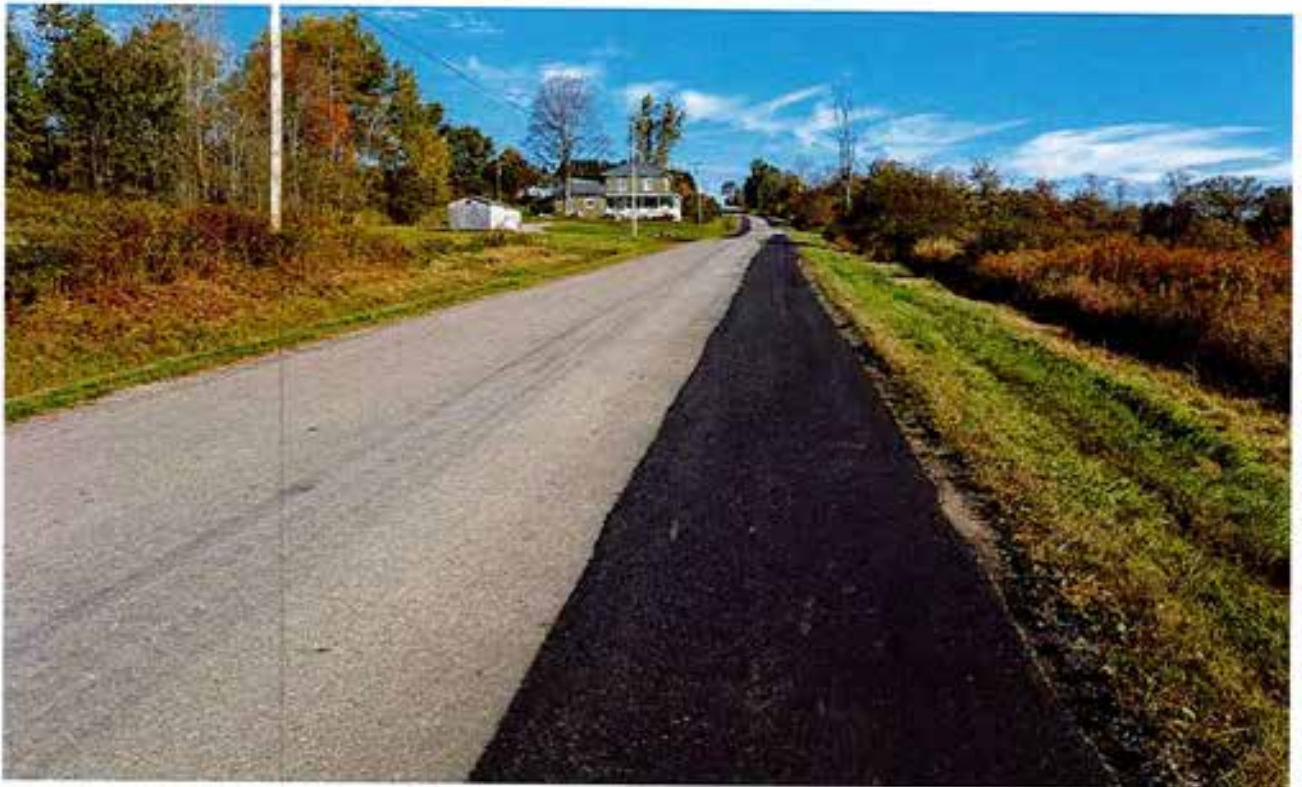
East edge of North Road (REPAIRED)
