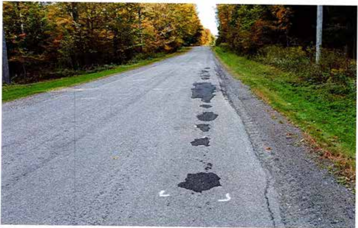
Eagle Street lane near 1000 (REPAIRED)
