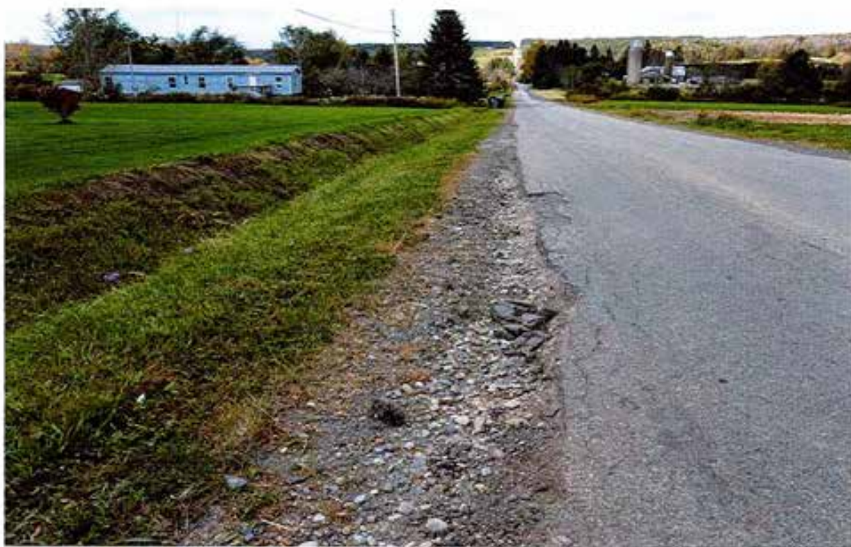
Bray Road South edge and shoulder near 409
