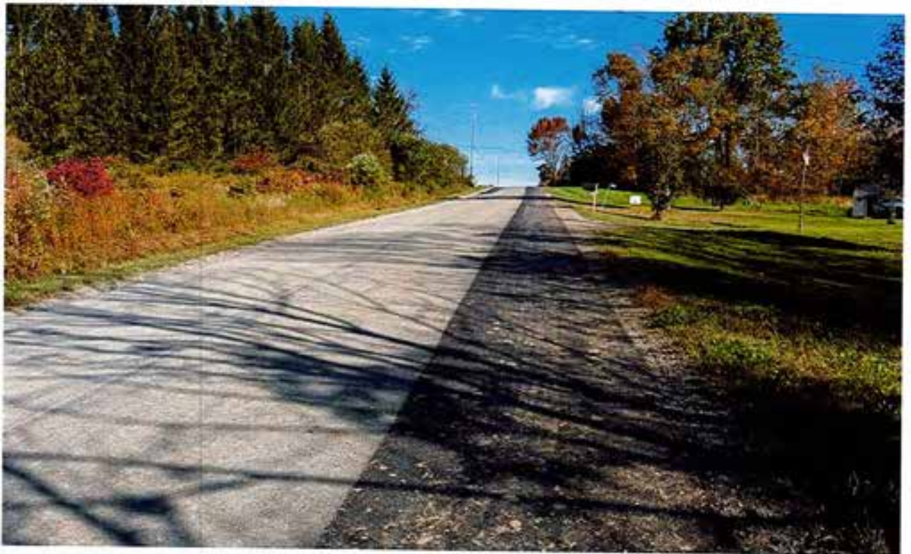
North Road East edge near 11582 (REPAIRED)
