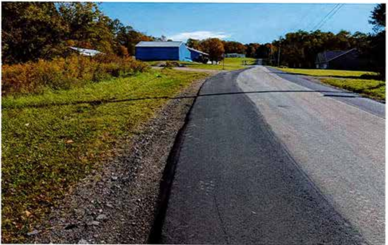
Eagle Street North and South side lane and edge near 1219 (REPAIRED)
