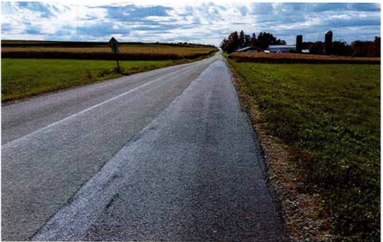
Brown Schoolhouse Road West shoulder from 11214 to 11123 (REPAIRED)
