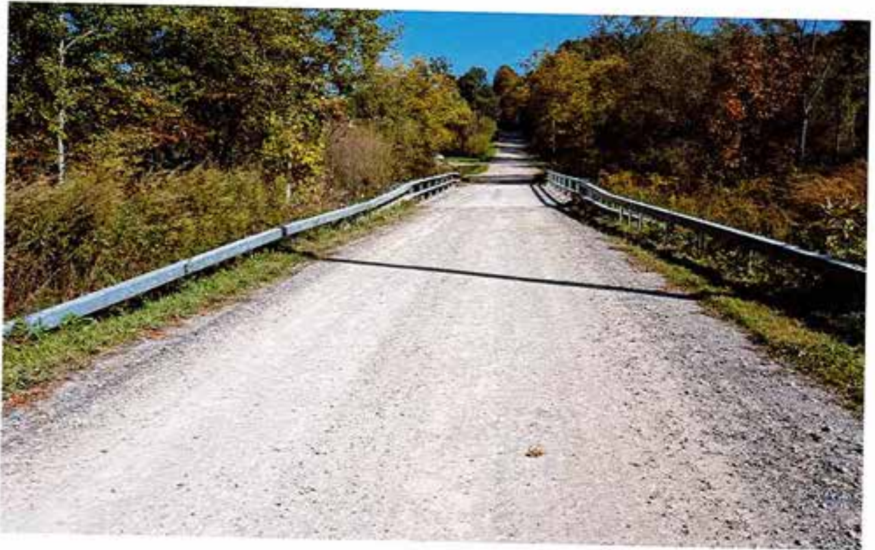
Jones Rd bridge
