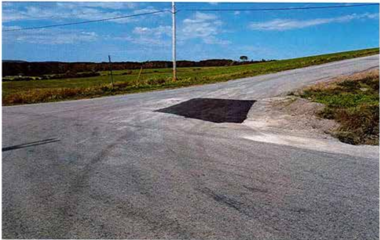
Edmunds Road intersection of Brown School House (REPAIRED)
