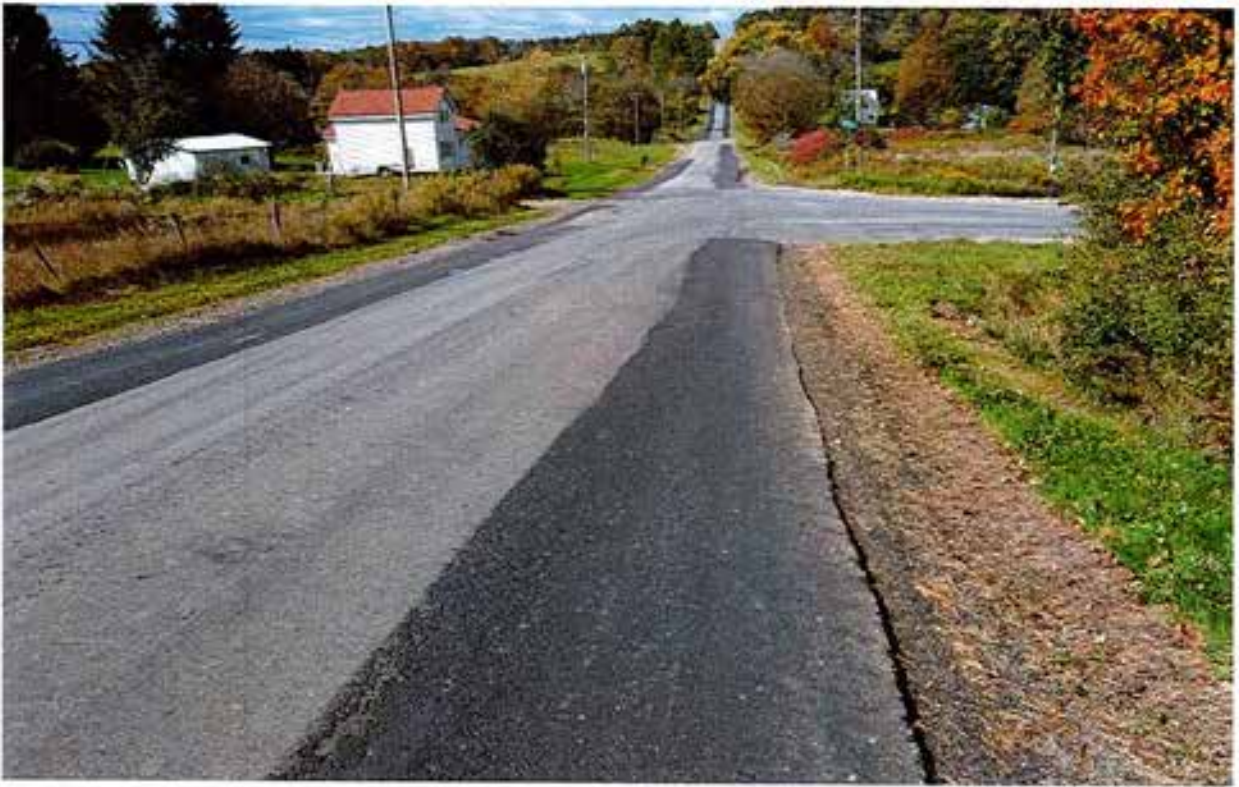
Bray Road North edge West of Hiram (REPAIRED)
