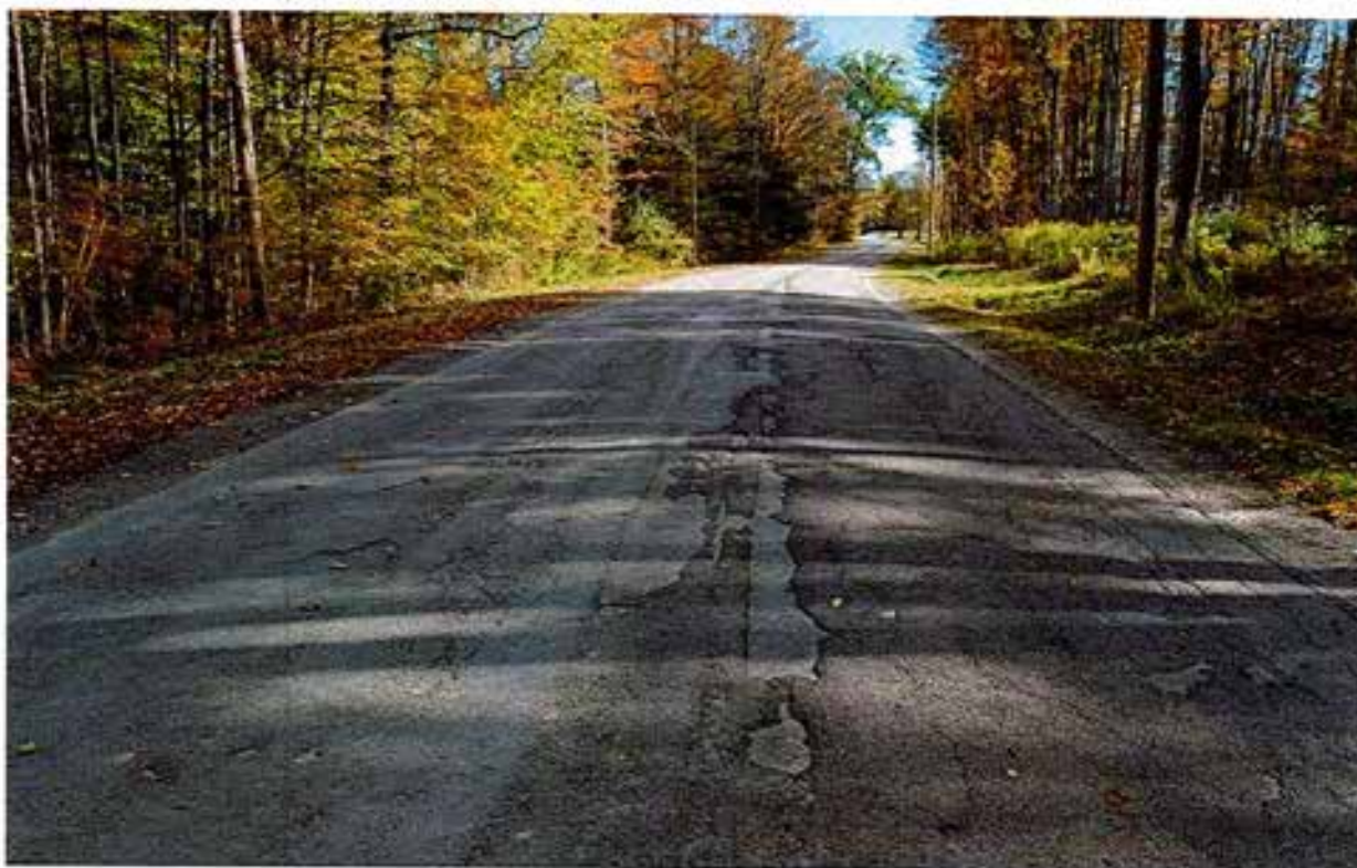
Eagle Street lane near 915
