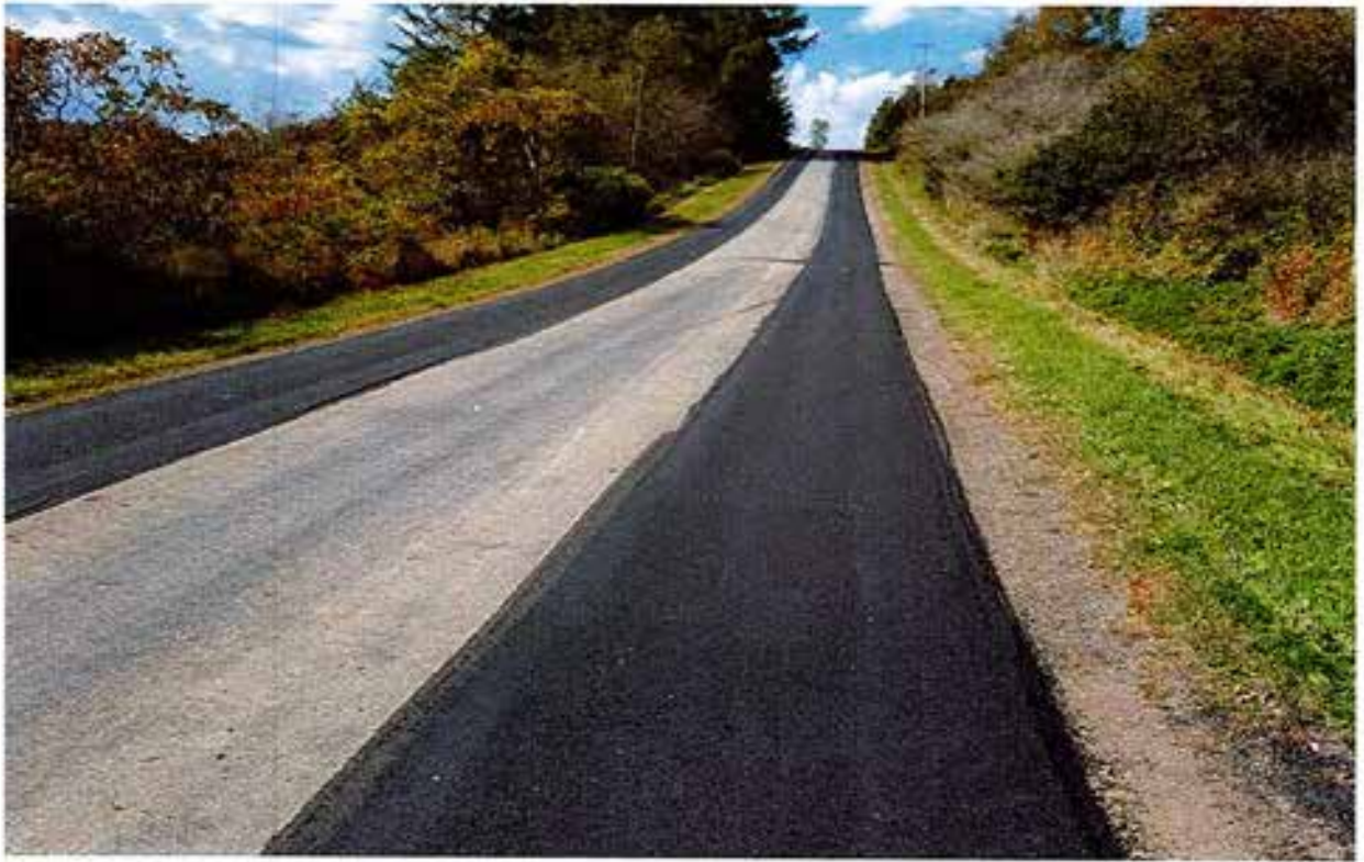
Bray Road North edge and shoulder from Eagle Street to +/- 2801 (REPAIRED)
