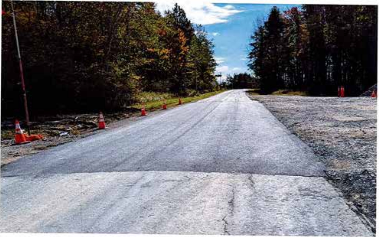
Galen Hill Rd pavement repair between construction entrances (REPAIRED)
