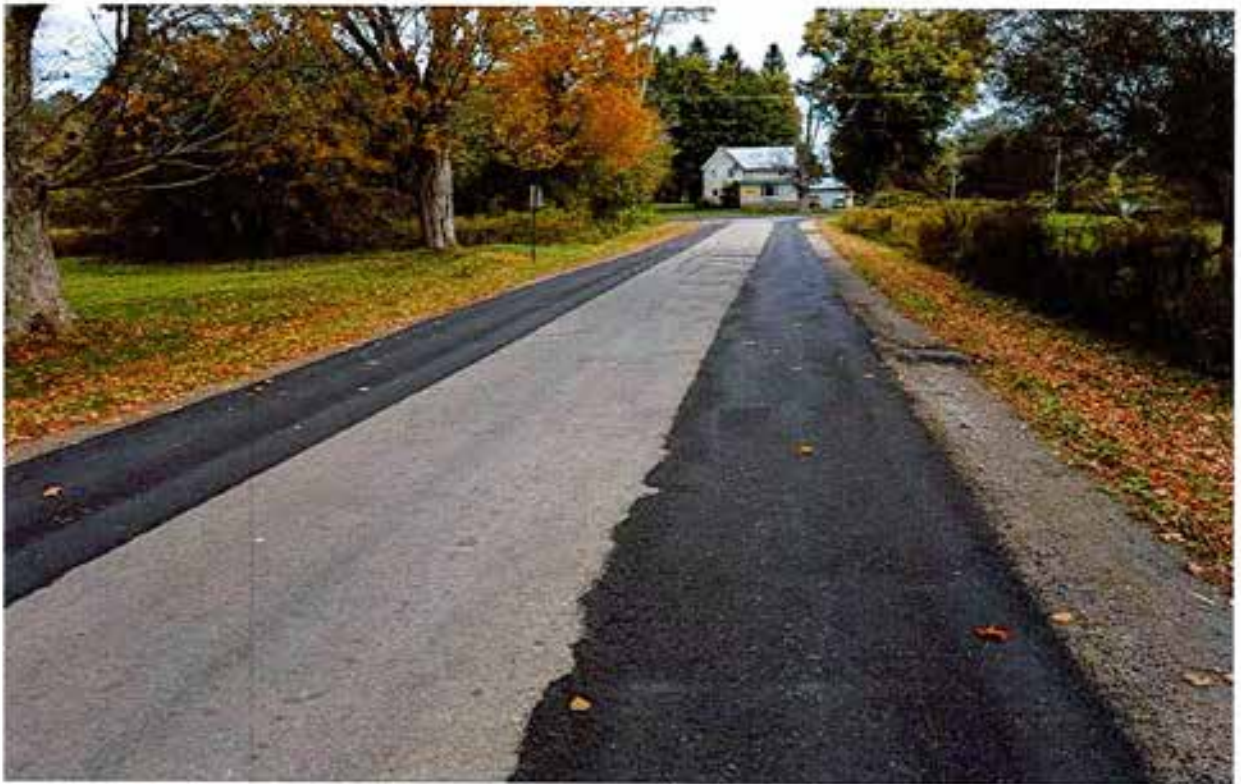
Eagle Street East lane near 708 (REPAIRED)
