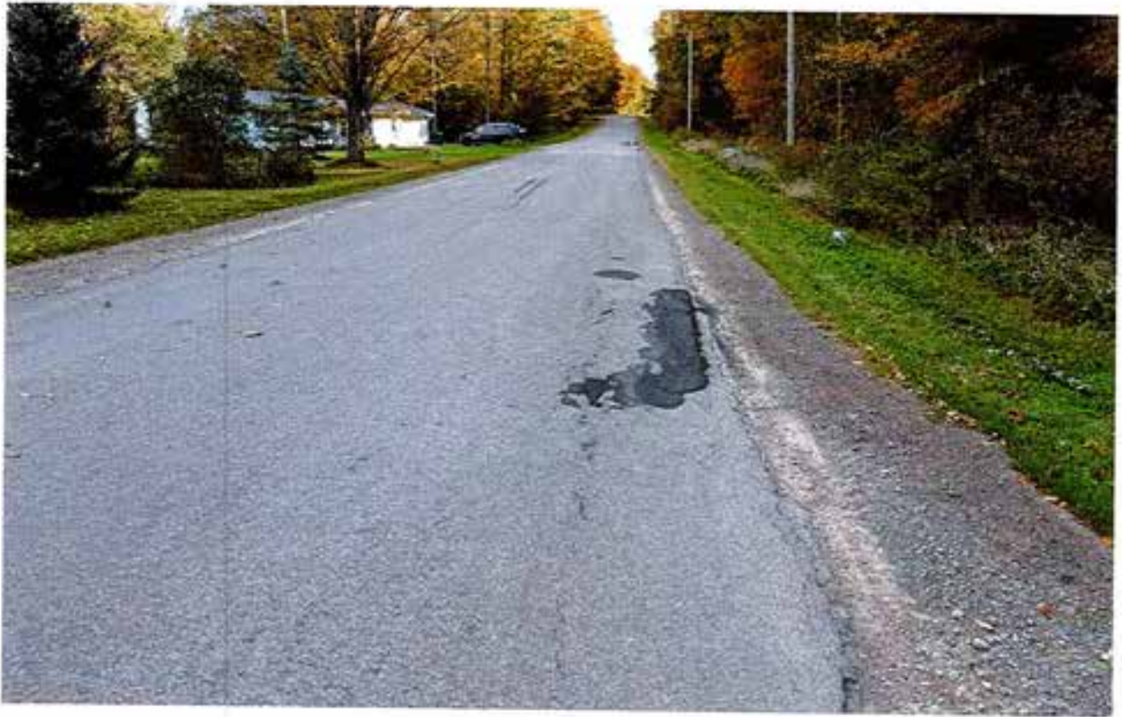
Eagle Street lane and East edge near 994 (REPAIRED)
