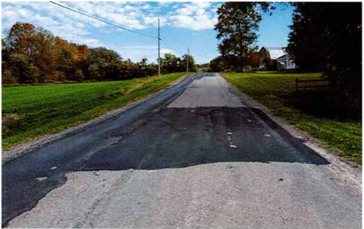
Eagle Street lane South of 849 (REPAIRED)
