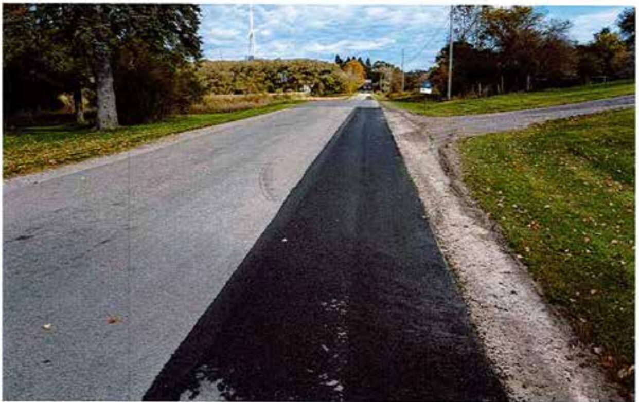
Eagle Street East edge and shoulder near 757 (REPAIRED)
