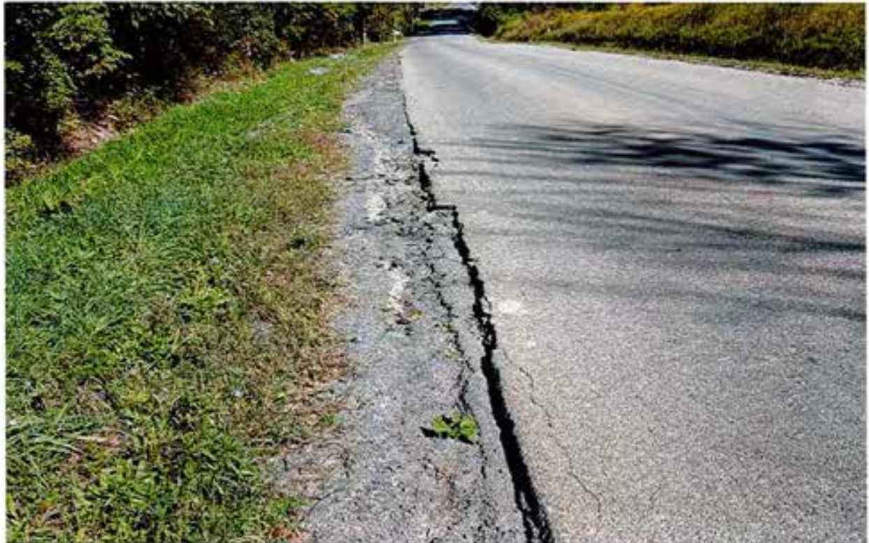
Brown Schoolhouse Road West shoulder North of 11448
