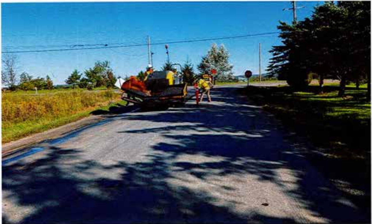
Lane deterioration North Rd near intersection with Bray Rd (REPAIRS IN PROGRESS)
