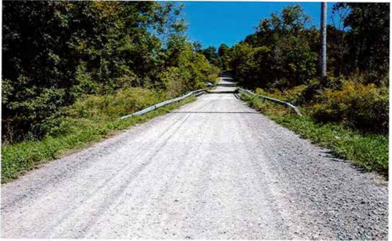
Jones Rd bridge
