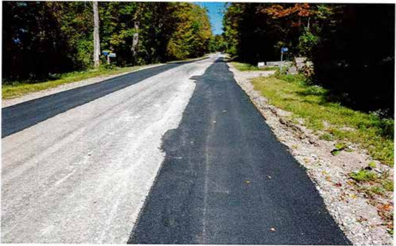
Osmun Road East lane and shoulder deterioration near 10200 (REPAIRED)
