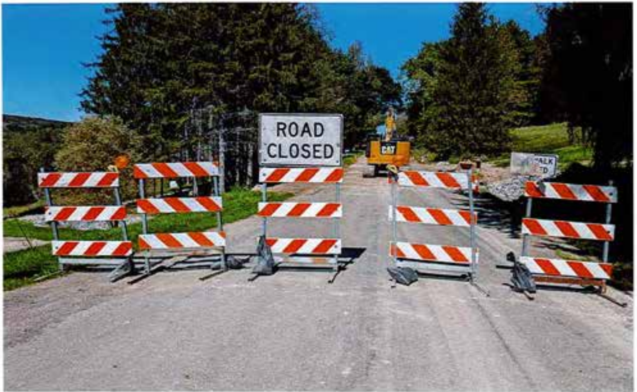
Osmun Rd: Road over Culvert near 10379 facing North (REPAIRS IN PROGRESS)
