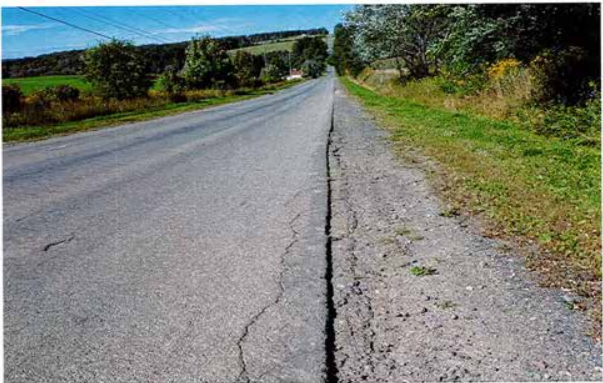
Bray Road North edge and shoulder deteriorating from 409 to 475
