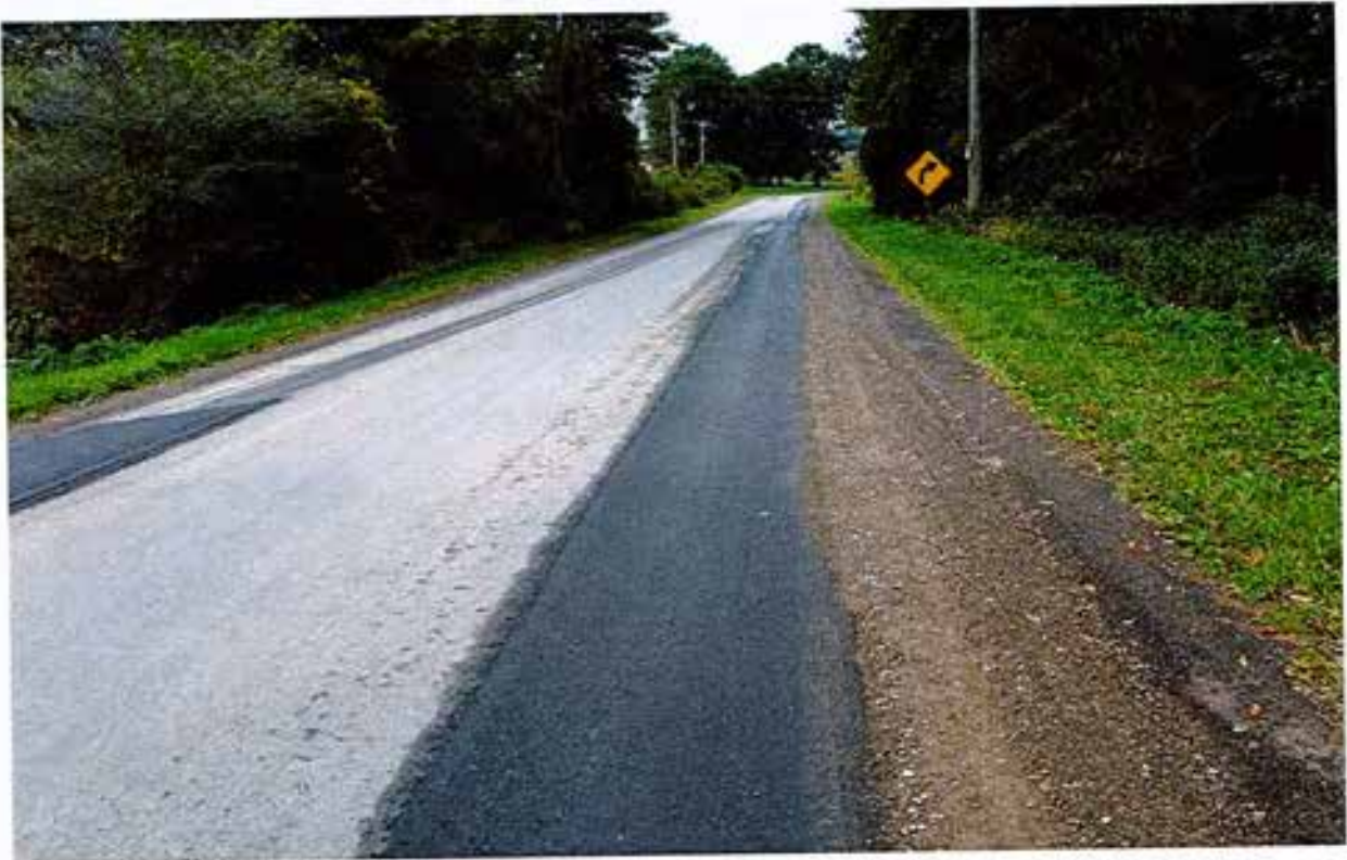
Siloam Road lane deterioration near intersection with Maple Grove (REPAIRED)
