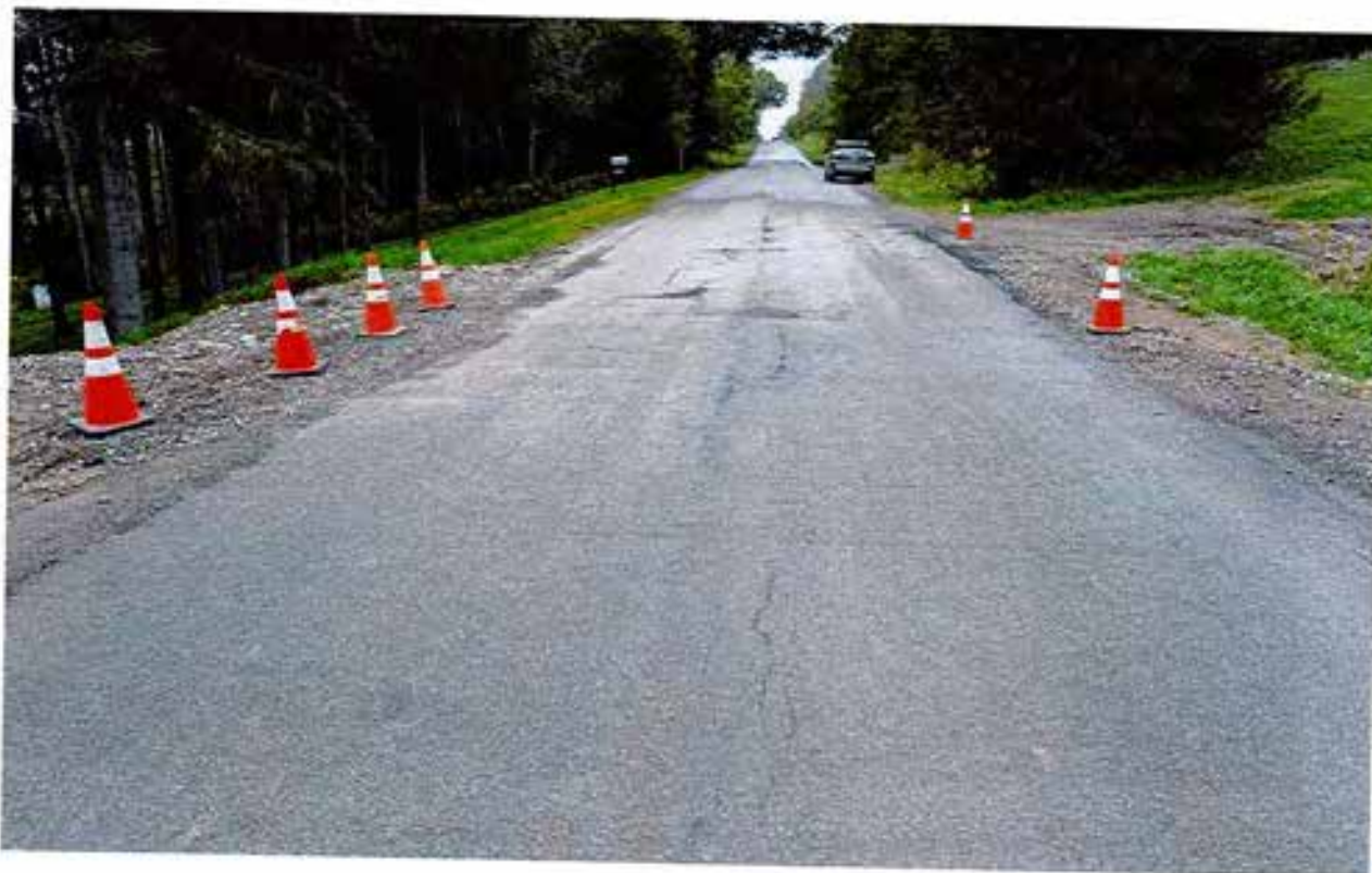
Osmun Rd: Road over Culvert near 10379 facing North
