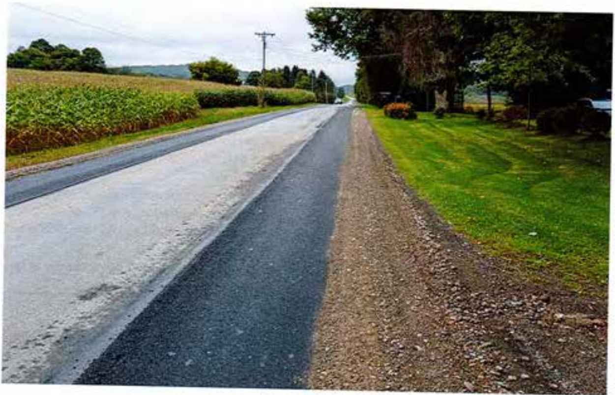
Siloam Road South shoulder deterioration near 1675 (REPAIRED)
