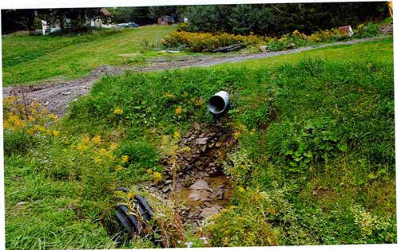
Osmun Rd: East side of 5' Dia. HDPE Culvert near 10379 facing East
