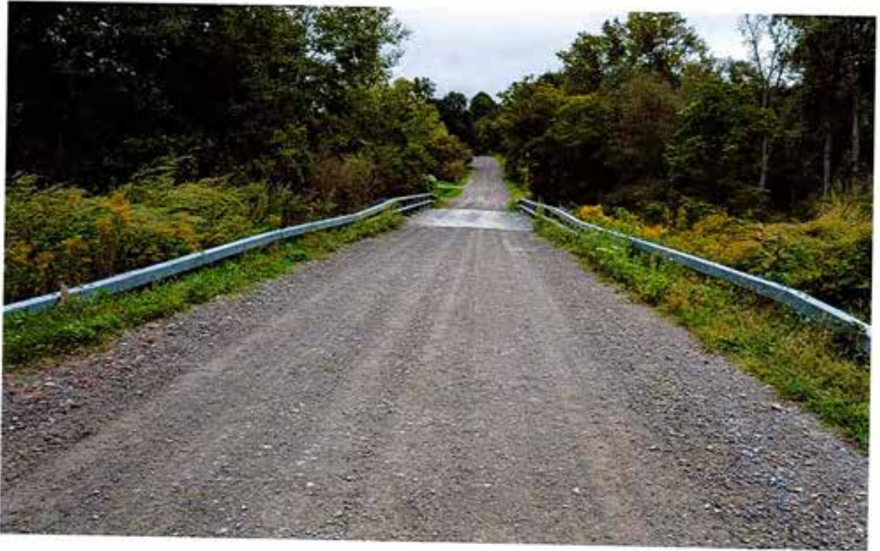
Jones Rd bridge
