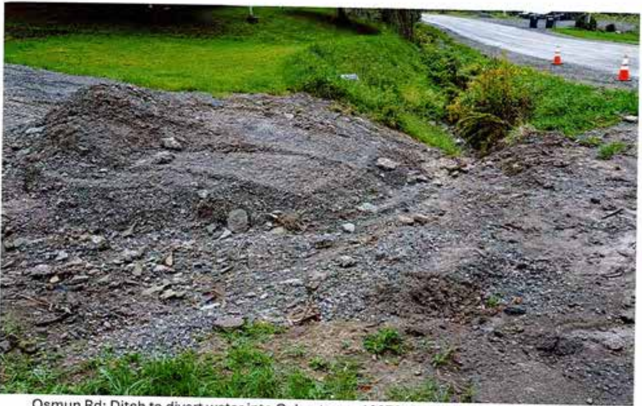
Osmun Rd: Ditch to divert water into Culvert near 10379. According to Town Highway Superintendent, the diversion ditch is helping prevent erosion. Ditch to be maintained as needed.
