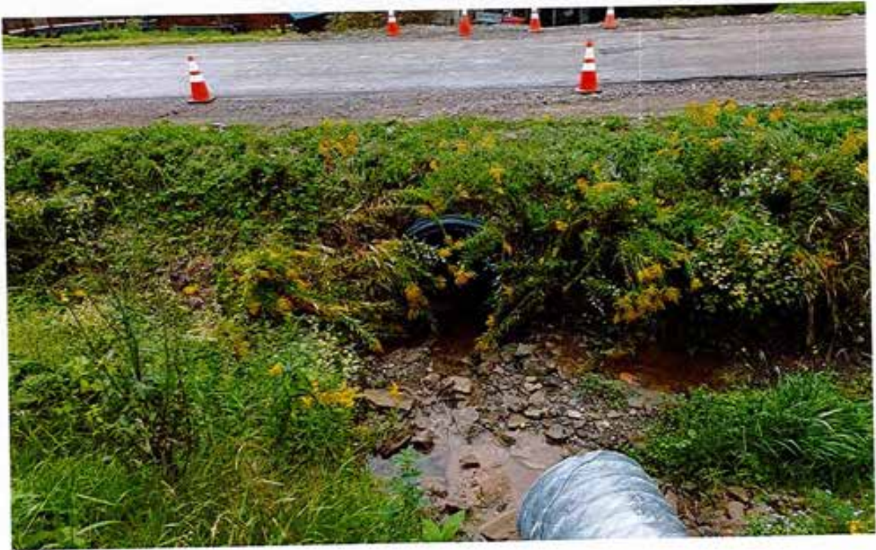
Osmun Rd: East end of 5' Dia. HDPE Culvert under Osmun Rd near 10379
