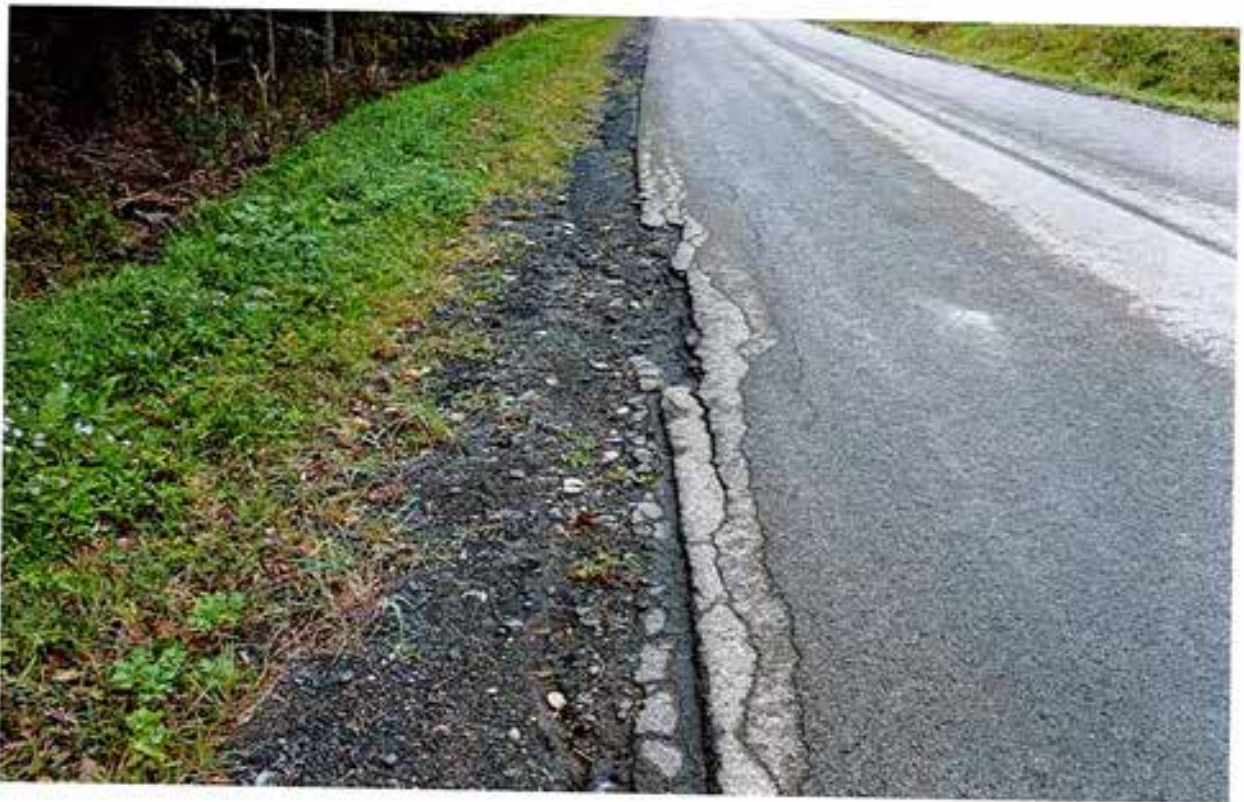
Brown Schoolhouse Road West shoulder North of 11448
