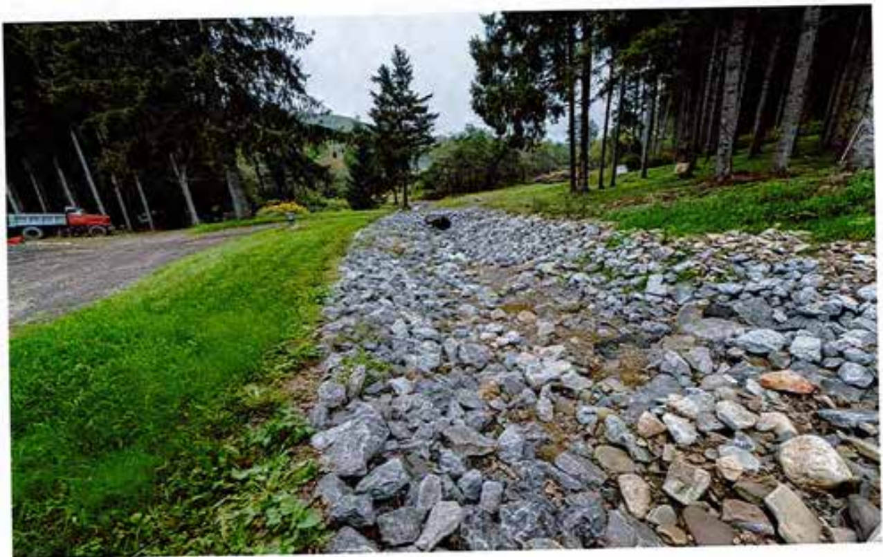
Osmun Rd: West side of Culvert near 10379 facing West
