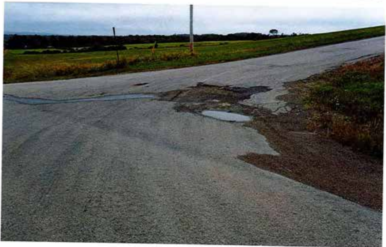
Edmunds Road intersection of Brown School House
