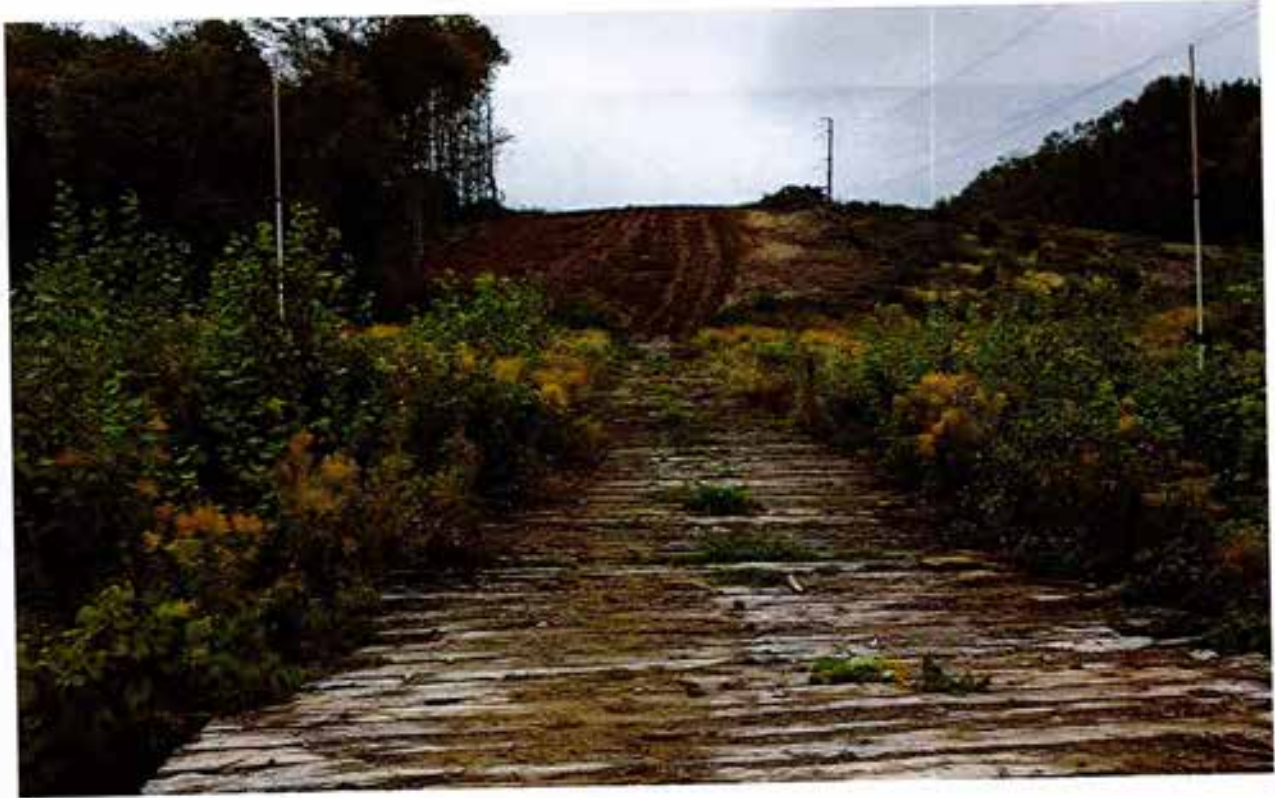
Osmun Rd: Construction Entrance nearest to Culvert @ 10379 facing East
